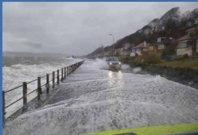
Figure 5. Coastal flooding on the A78 South West Scotland, 3rd Jan 2014 (photo from Scotland TranServ)
