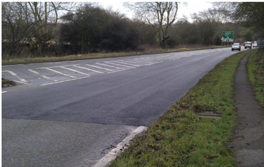
**Figure 3-9: HMA section and boundary to pre-existing surface (bottom-left)**
