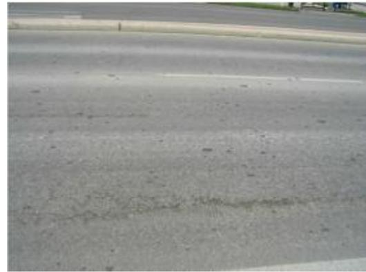
**Figure G-14: Evidence of cracking in both WMA and HMA sections**
