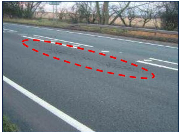
**Figure B-8: T crack in SB lane (Section 1900A5/171, ch. 0 m)**
