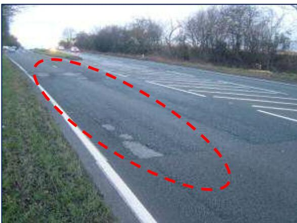
**Figure B-15: L crack in OS edge of SB lane (Section 1900A5/157, ch. 0 m)**
