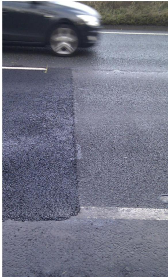
**Figure 3-7: Boundary of the LTA (left) with the existing surface (right)**
