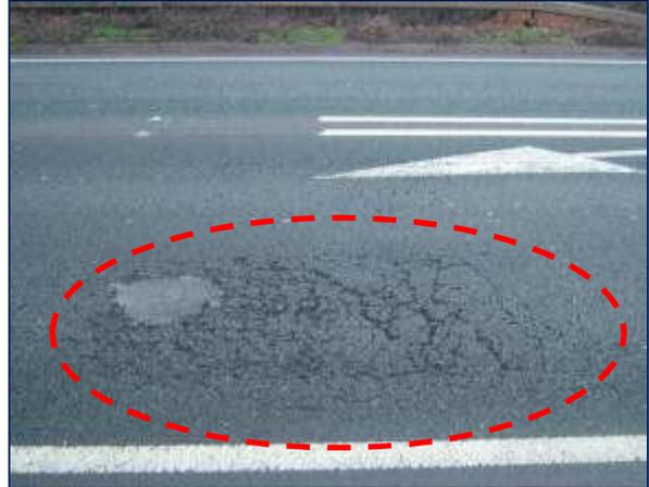
**Figure B-6: L+T cracks in SB lane (Section 1900A5/171, ch. 0 m)**
