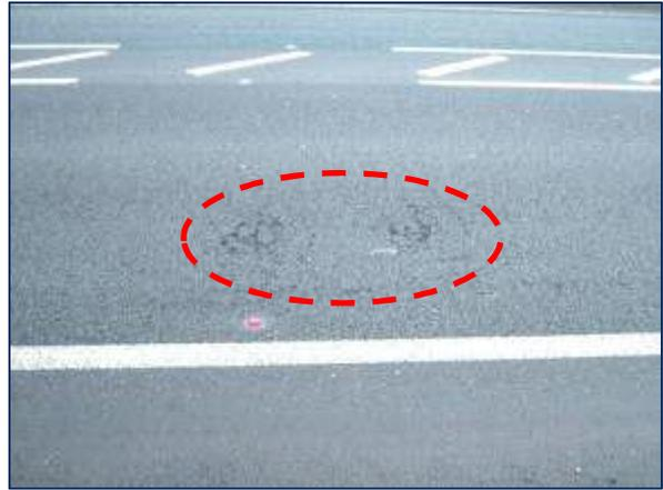
**Figure B-12: L+T cracks (NB lane) 2230 (Section 1900A5/157, ch. 39 m)**
