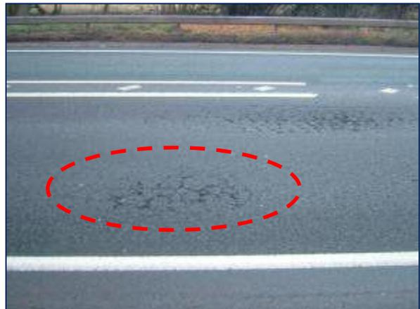
**Figure B-10: Transverse cracks (NB lane) (Section 1900A5/157, ch. 17 m)**
