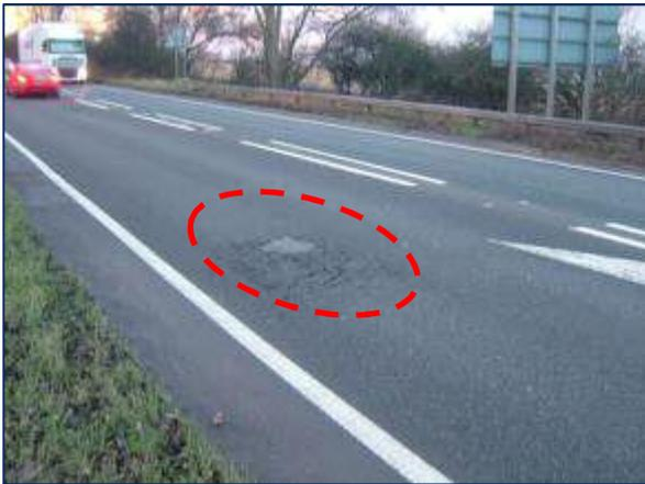
**Figure B-7: General SB view - poor surface dressing (Section 1900A5/171, ch. 0 m)**
