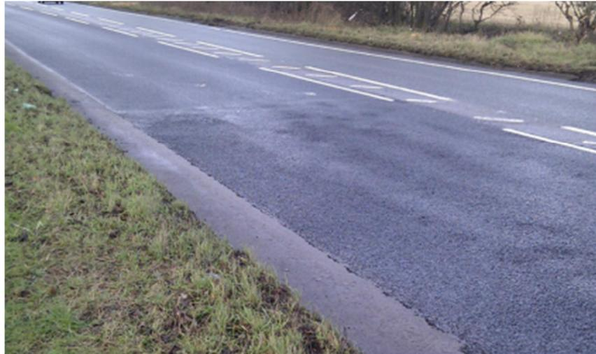
**Figure 3-8: Boundary between new LTA and HMA mixtures**
