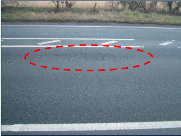
**Figure B-11: T cracks (NB lane) 2229 (Section 1900A5/157, ch. 25 m)**
