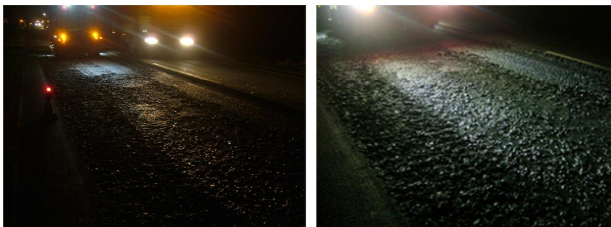
**Figure 3-5: Photographs taken after planing in the section to be inlaid with LTA mixture**
