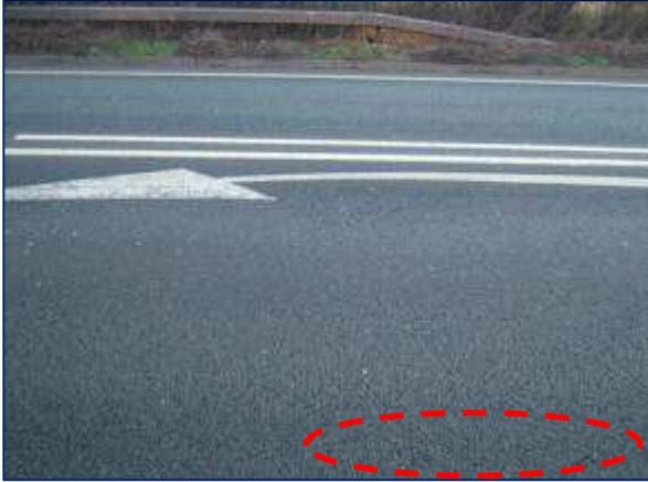
**Figure B-5: L crack(s) in OS edge of SB lane (Section 1900A5/171, ch. 0 m)**
