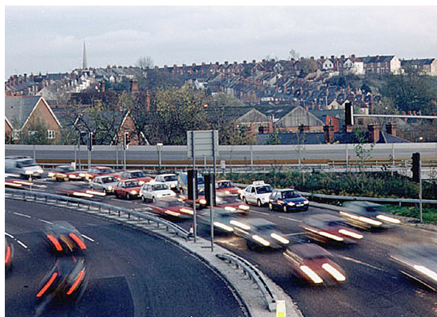
Figure 1 Long-life asphalt roads cope with higher traffic levels
