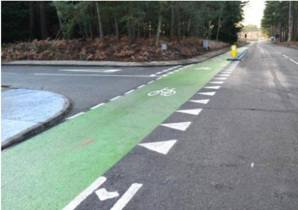
**Figure 2: Cycle lane marked across the junction using triangular markings**
