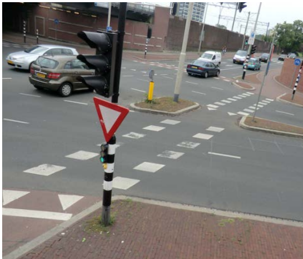
Figure 5 - Different stop line locations for cyclists and motor vehicles also illustrating the use of Elephant feet and Sharks teeth road markings (Source:
