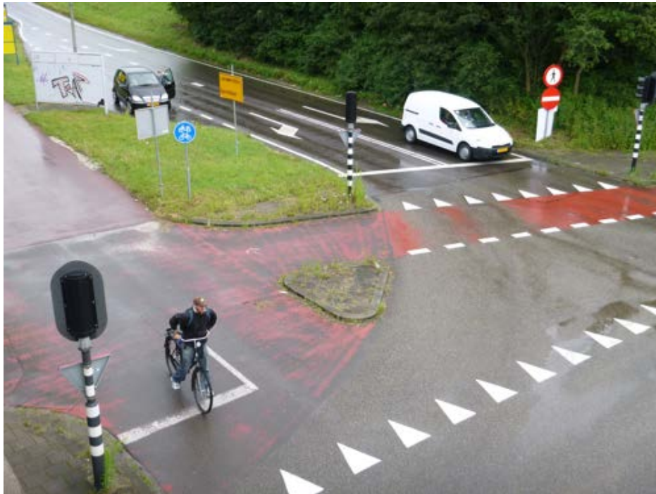
Figure 4 – photograph of a junction showing separation between bicycle stop line and the motorised traffic stop line.
