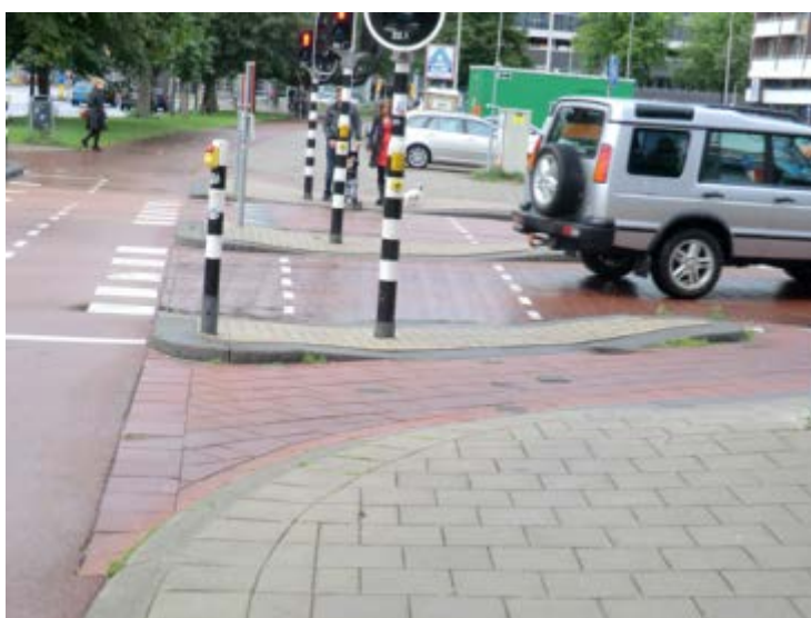
Figure 3- Photograph of a pedestrian platform
