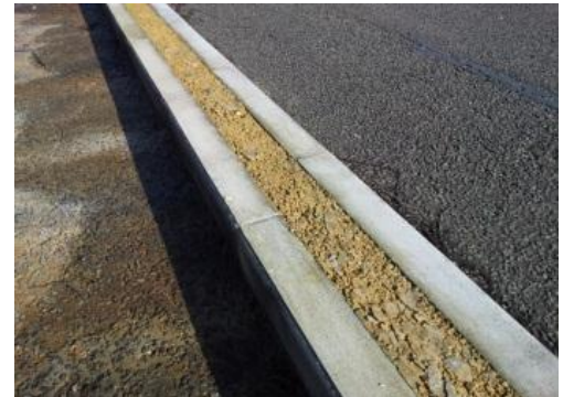
A kerb with a 365 mm hard margin
