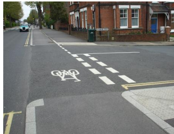
Raised cycle track crossing side-road, Brighton
