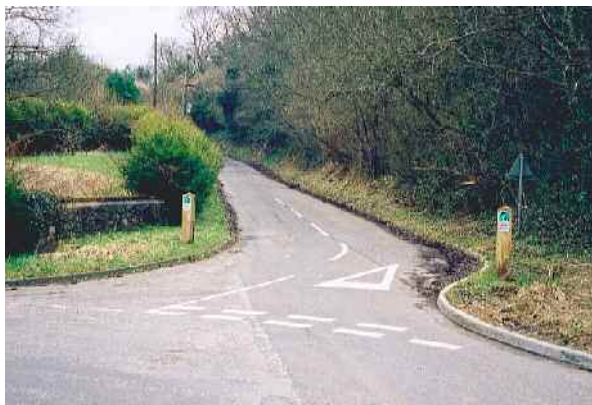
Figure 5: Signing arrangement at entrance to Quiet Lane
