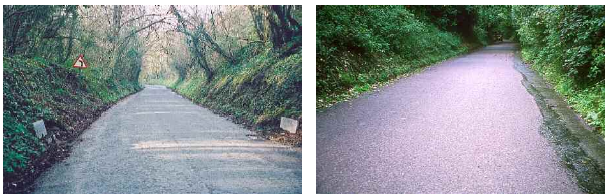
Figure 8: Thong Lane – before (left) and after pink surface dressing (right), leaving the edges of the road unchanged, to make the road appear narrower.
