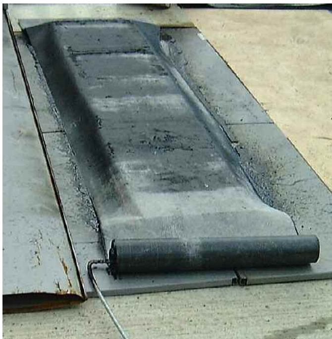
(c) Membrane immediately after application
