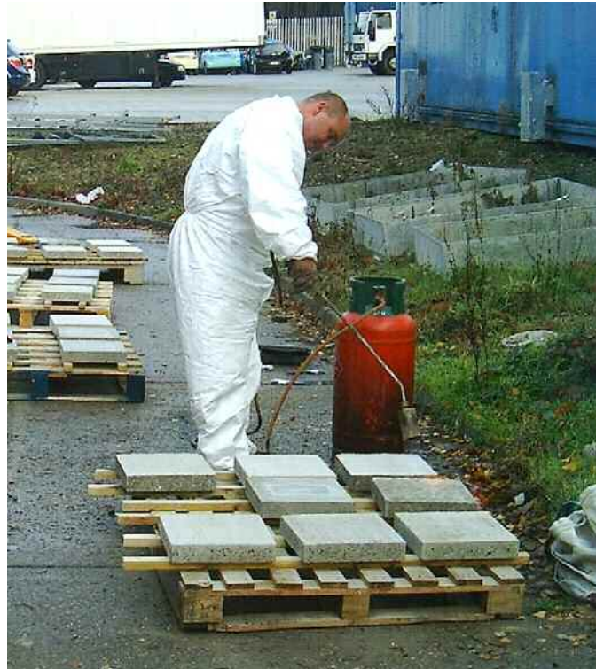
Figure 2. Drying the slabs prior to the application of the primer
