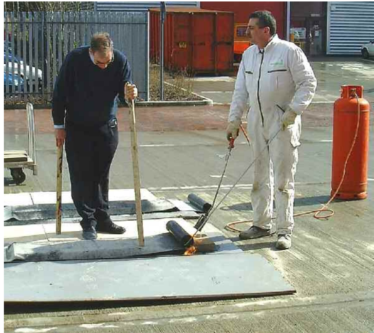
(b) Torching-on the membrane
