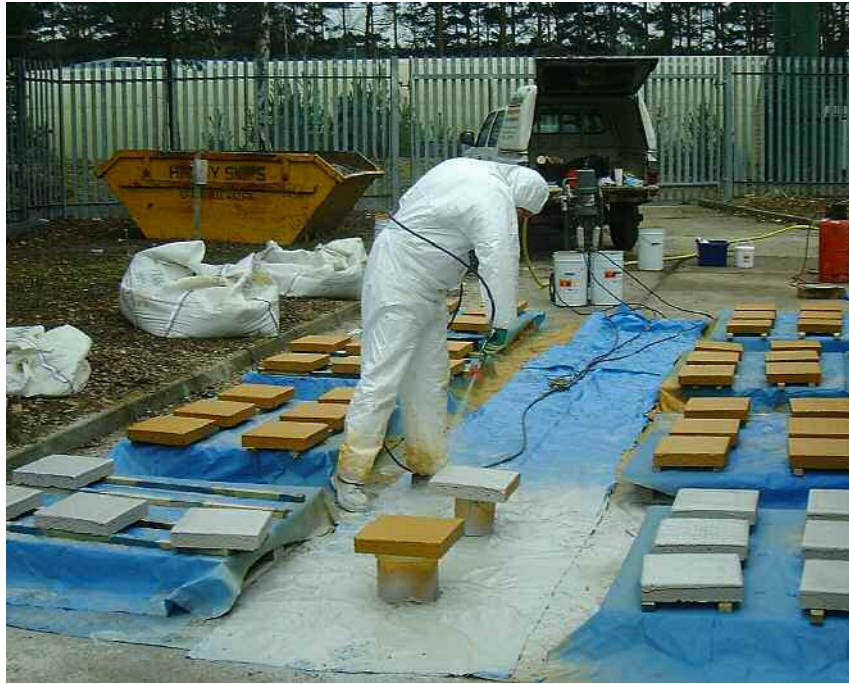
Figure 3. Application of the second coat of a spray applied waterproofing membrane
