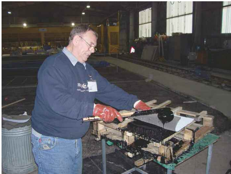
Figure 4. Application of sheet waterproofing membrane
