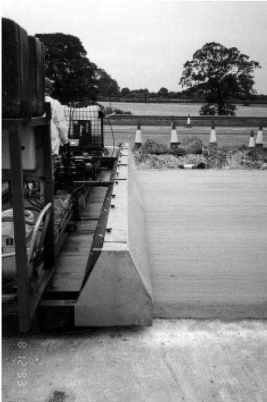
**Plate 1** Application of the retarder to the fresh concrete surface
