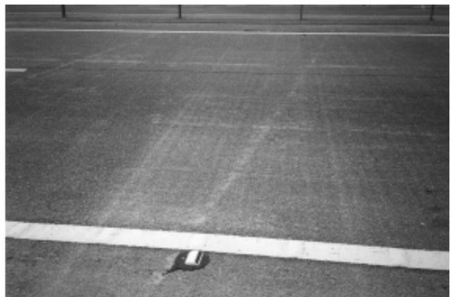
**Plate 7** Diagonal ridges on road surface left by super-smoother
