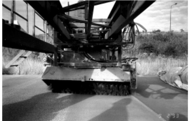
**Plate 3** Action of the brush used to expose the surface of the concrete
