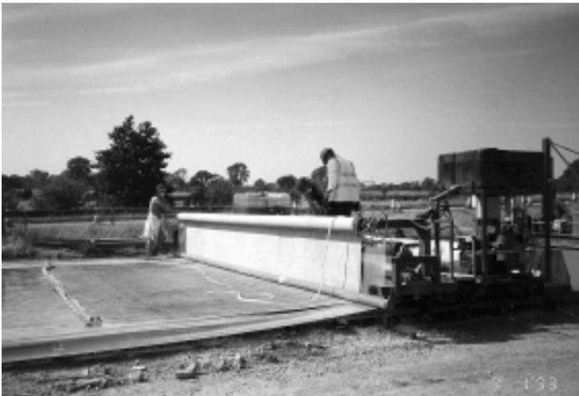
**Plate 2** Application of polythene sheet (after retarder has been applied)
