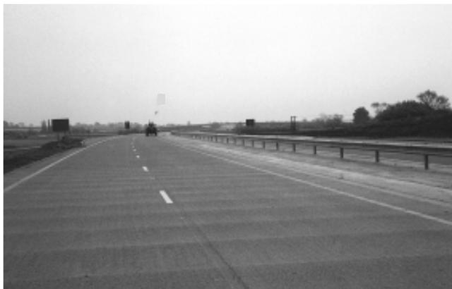
**Plate 8** Transverse stripes across the road as a result of brushing the exposed aggregate surface
