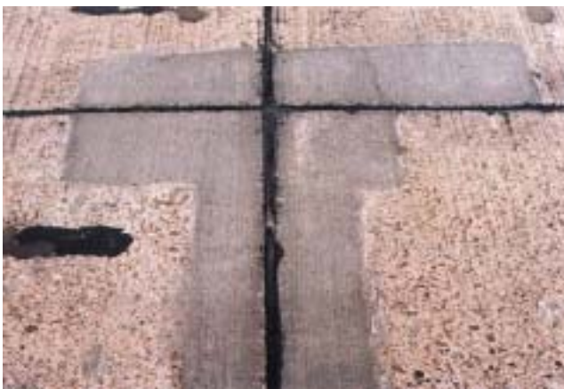
Plate 8 Air entrained concrete (M11)
