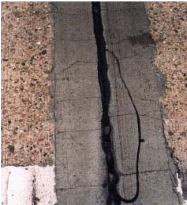
Plate 3 SBR mortar (M11)
