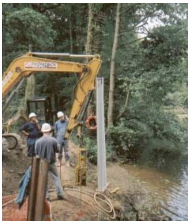
**Figure B1** Driving plastic sheet piles at Vann Lake
