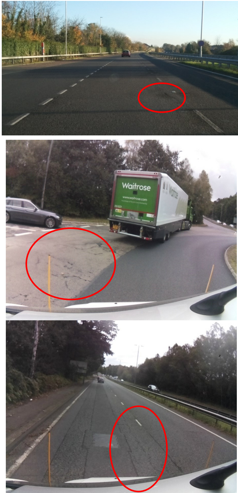
Figure 5: Images from PiCam taken on the A3095 and A329(m) with defects highlighted
