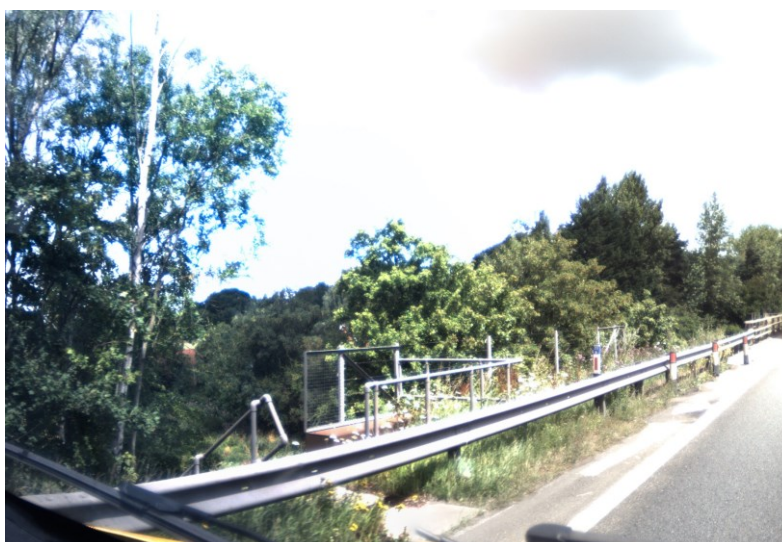
Figure 6-5: View from the M5 carriageway showing top of bridge/embankment access stairs
