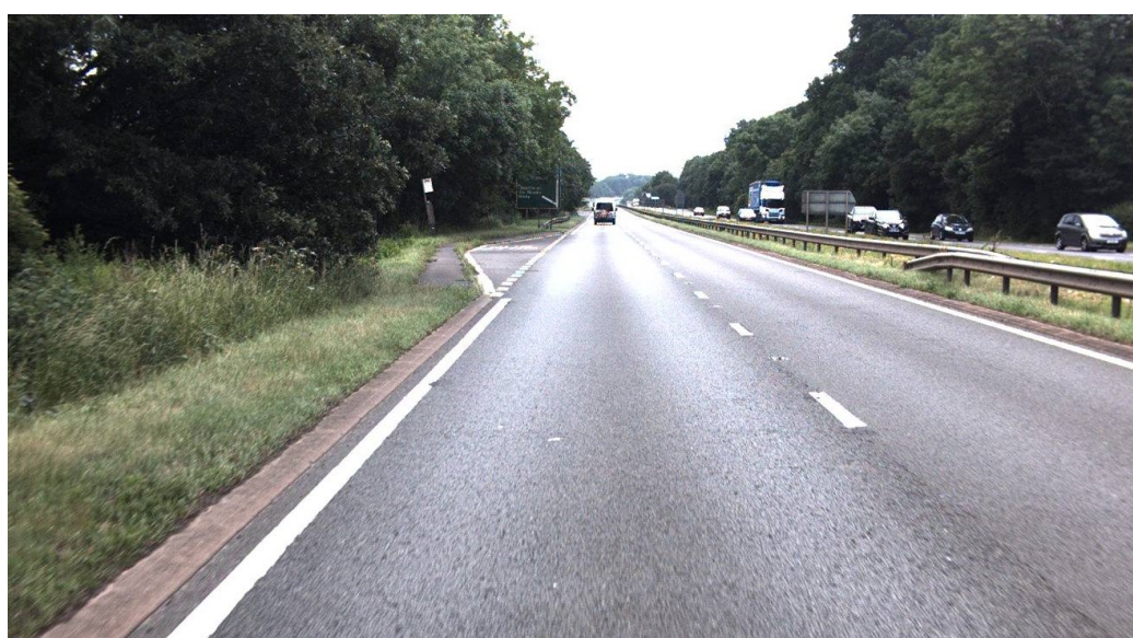
Figure 6-7: Photo of the location of the cluster of slip events near a bus stop and footpath crossing on the A46 north of Syston
