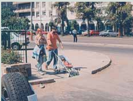
Figure 2.9 Provision of kerb ramps benefit all users
