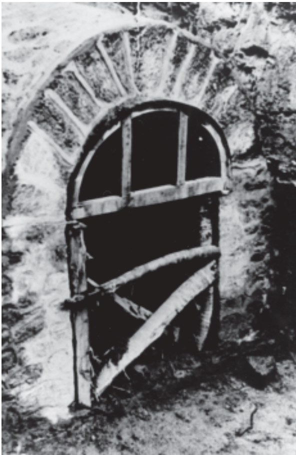
Figure 15.5 Masonry arch culvert with simple wooden formwork
