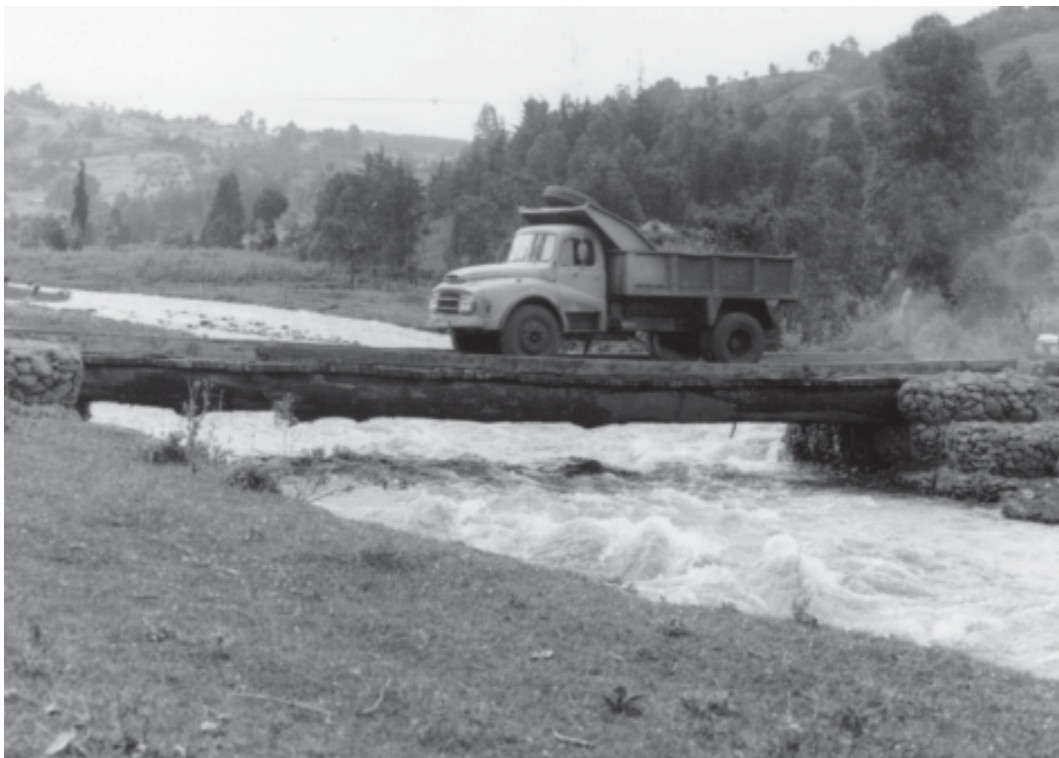
Figure 13.3 Temporary bridge on gabion abutments
