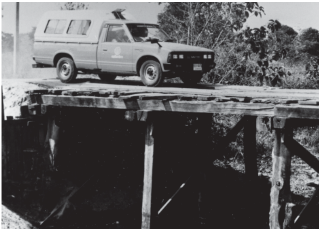
Figure 13.6 Timber deck on piled piers and abutments
