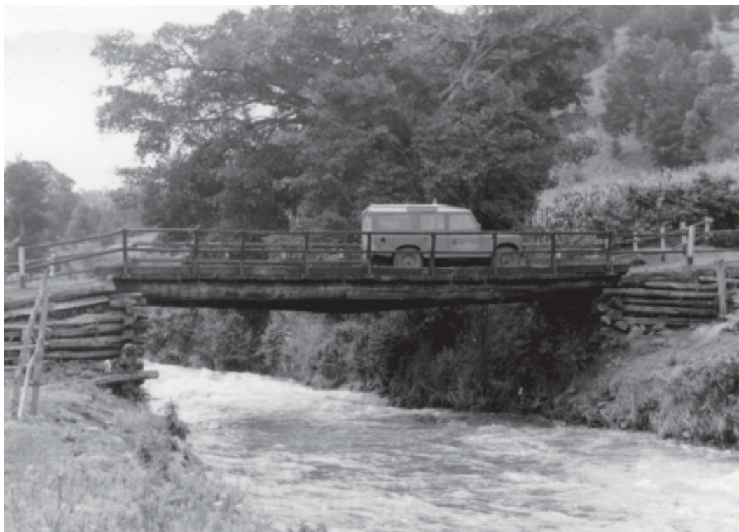
Figure 13.4 Log abutments with integral wing walls
