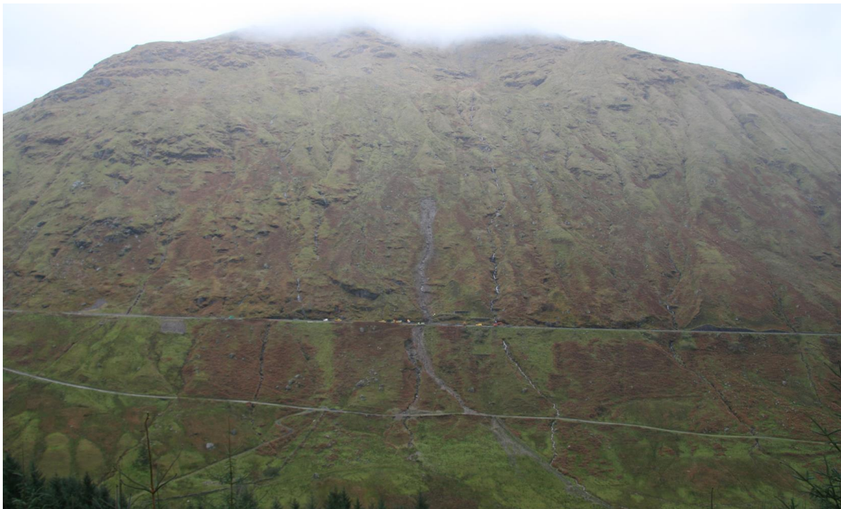
Figure 2.2: View of the hillside above and below the approach to the Rest and be Thankful from the east (from NGR NN 23160 06559 on the opposite side of Glen Croe). Not only can the event dated 28 October 2007 be clearly seen but evidence of numerous past events can be seen on the surrounding hillside
