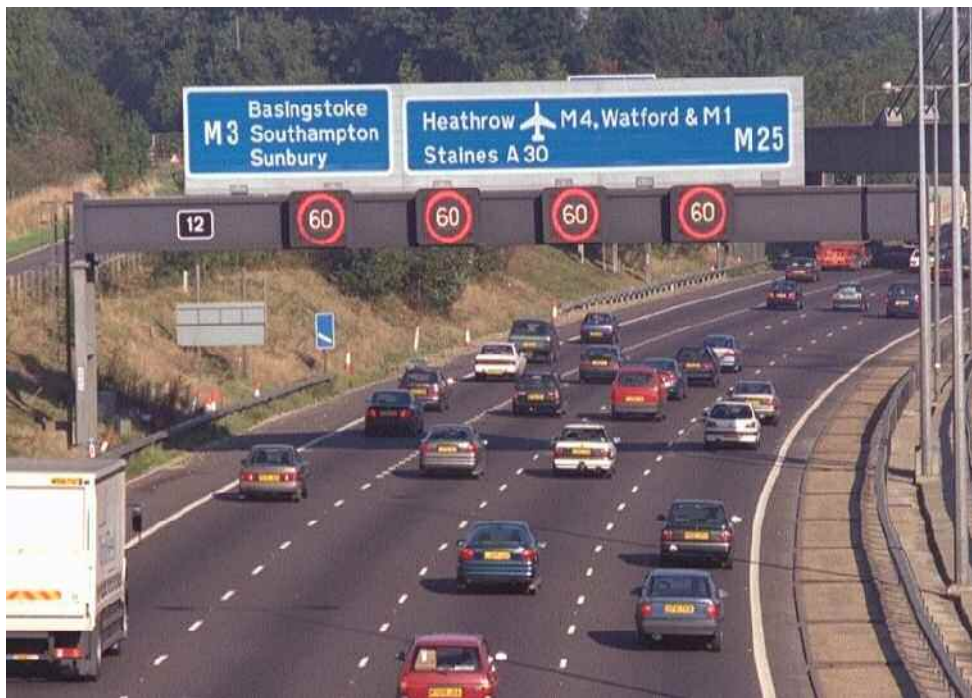
Figure 1.1.1 - The Controlled Motorways Environment
