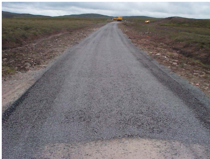
Figure 2.5 – The completed tyre bale road construction on the B871. (Photograph © Highland Council.)
