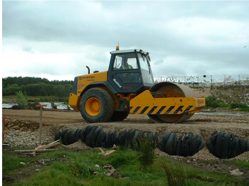
Figure 4.2 – Construction of the landfill access road. (Photograph © Northern Tyre Recycling.)
