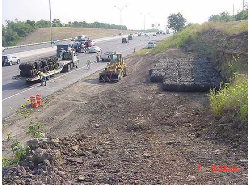
Figure 5.3 – Placing tyre bale layer two in the excavated IH30 slope failure, note the cover to layer one. (Photograph © Texas Department of Transportation.)
