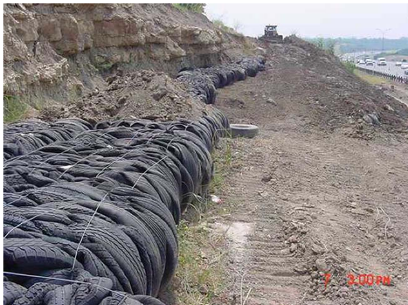
Figure 5.4 – Placing tyre bale layer three in the excavated IH30 slope failure, note the cover to layers one and two. (Photograph © Texas Department of Transportation.)
