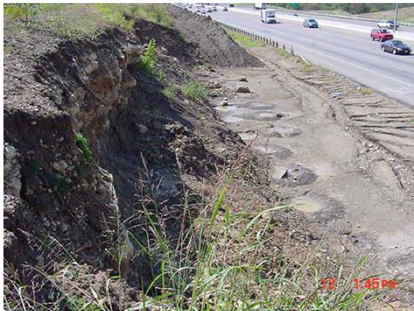
Figure 5.1 – The IH30 slope failure after excavation of the failed material. (Photograph © Texas Department of Transportation.)
