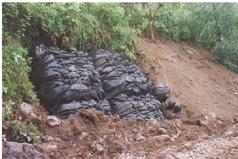
Figure 7.2 – Construction of the slope repair. (Photograph © Northern Tyre Recycling.)
