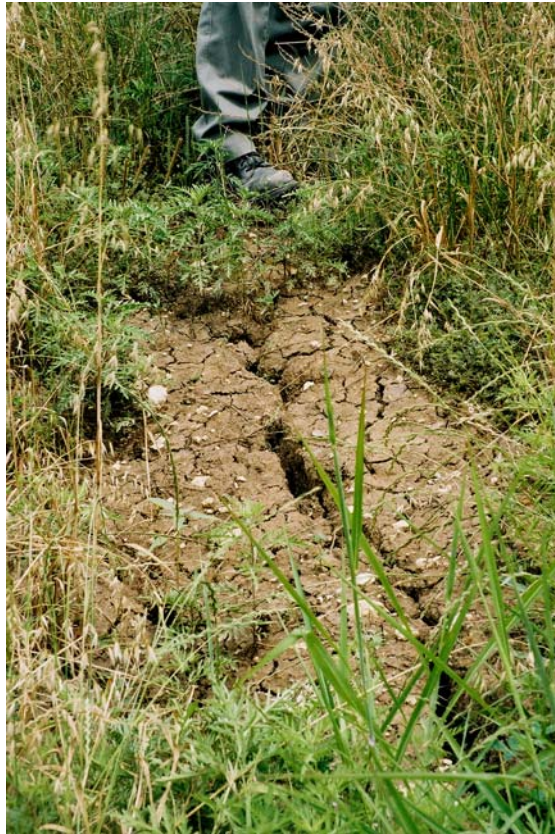
Figure 5.9 – Cracks at the crest of the slope in May 2004, demonstrating potential for further failure in the upper part of the slope which was backfilled with in-situ soil rather than tyre bales.
