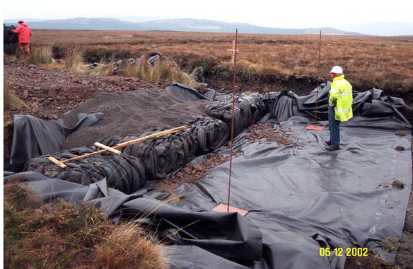
Figure 2.3 – Tyre bale construction on the B871 showing the settlement rods. (Photograph © Highland Council.)
