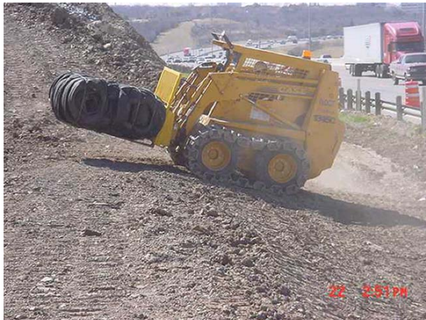
Figure 5.5 – Moving tyre bales up the partially constructed slope repair to layer three. (Photograph © Texas Department of Transportation.)
