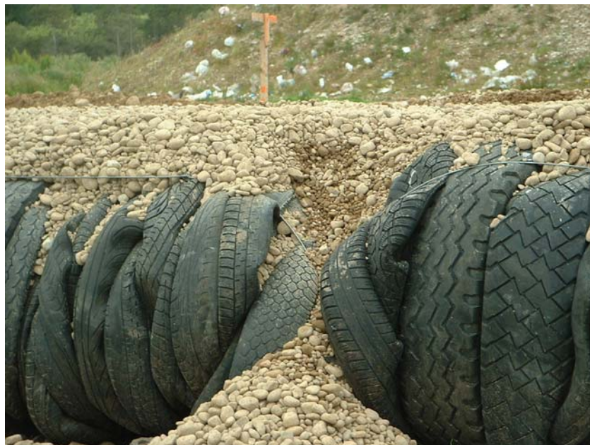
Figure 4.3 – Detail of the constructed landfill access road. (Photograph © Northern Tyre Recycling.)
