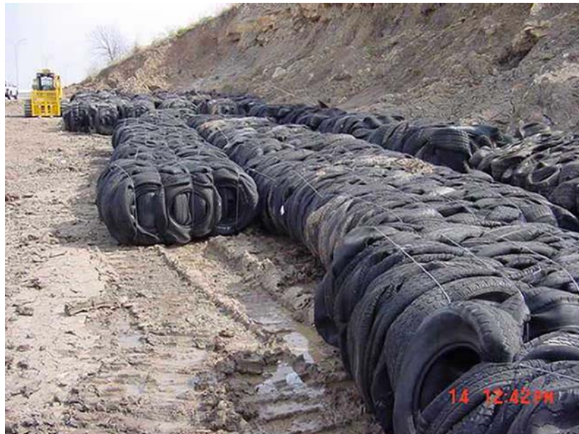
Figure 5.2 – Placing tyre bale layer one in the excavated IH30 slope failure. (Photograph © Texas Department of Transportation.)
