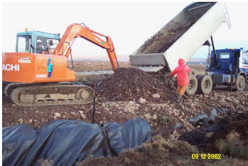
Figure 2.4 – Road construction on top of the tyre bales on the B871. (Photograph © Highland Council.)
