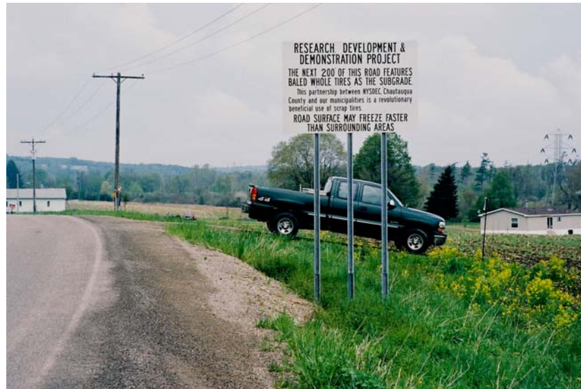
Figure 1.6 – Tyre bale section of CR342. The warning signs regarding the potential for early freezing are likely to be removed in the near future.
