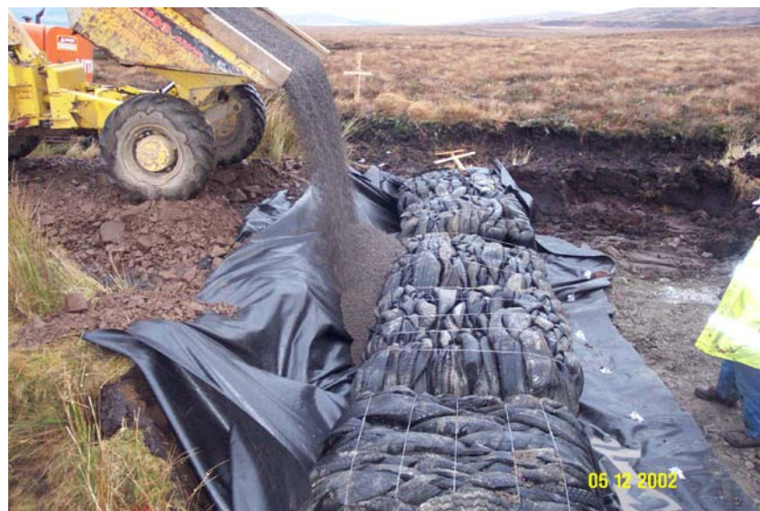
Figure 2.2 – Placing the tyre bale infill on the B871. (Photograph © Highland Council.)
