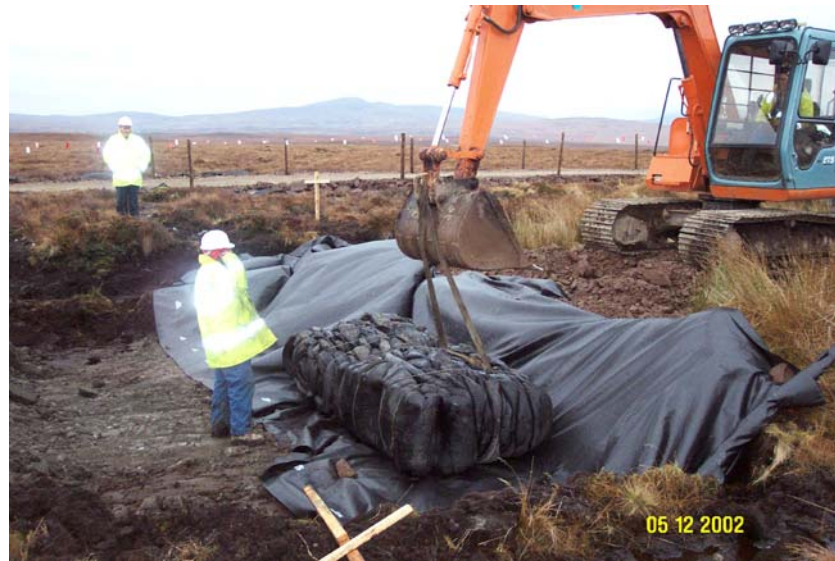
Figure 2.1 – Placing the tyre bales on the B871. (Photograph © Highland Council.)
