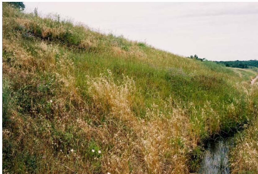
Figure 5.8 – Water drained to the front face of the slope by layers one and two of the tyre bales, May 2004.
