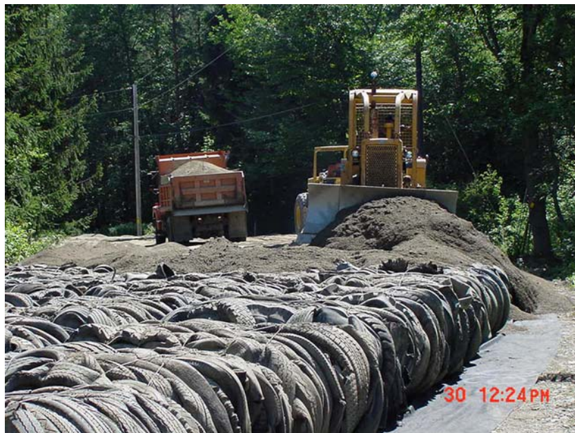
Figure 1.4 – Construction of the tyre bale section of CR342 – placement of the sand layer. (Photograph © Chautauqua County Department of Public Facilities.)
