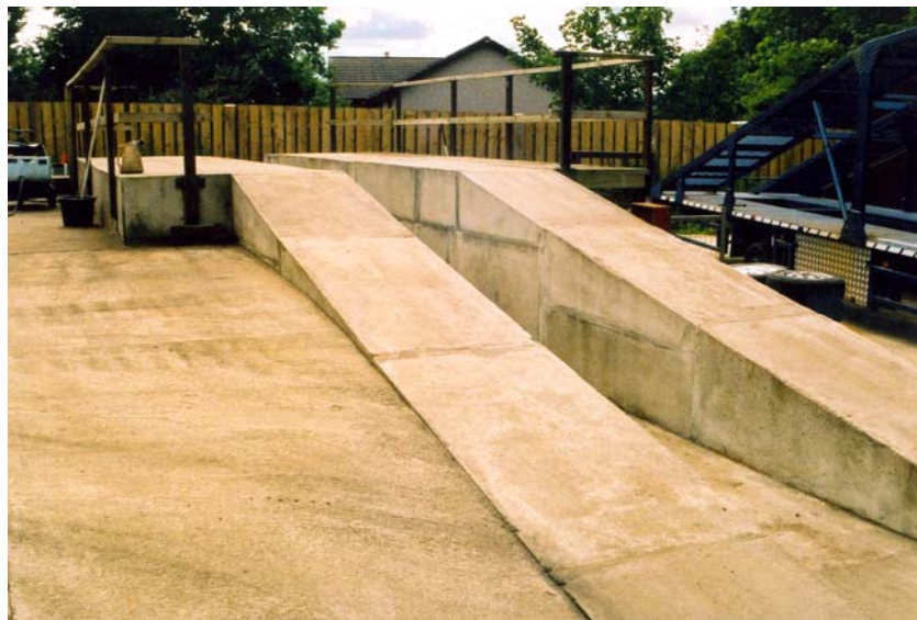
Figure 9.3 – The completed vehicle ramp constructed from concrete tyre bale blocks.
