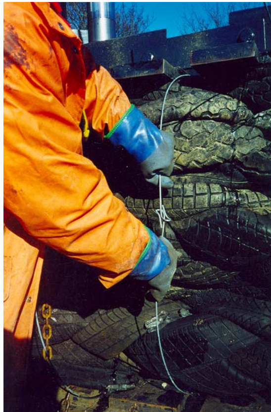
Figure B.5 – Connecting the Jamlock TM loops of the tie-wires together. (Photograph © Northern Tyre Recycling Ltd.)
