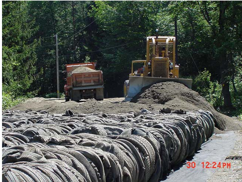
Figure 5.3 – Placing material to fill the voids between the bales. (Photograph © Chautauqua County Department of Public Facilities.)
