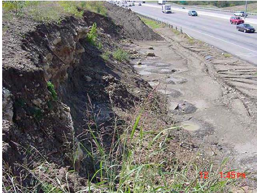
Figure 5.8 – Slope failure alongside Interstate Highway IH30 at Fort Worth, Texas. (Photograph © Texas Department of Transportation.)
