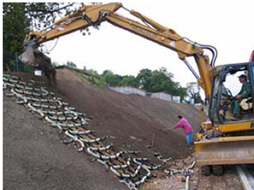
Figure 6.9 - Anti-erosion 'rope' geogrid for the promotion of vegetation growth on steep slopes developed by the Saxon Textile research Institute in Chemnitz, Germany ( http://www.tu-chemnitz.de/tu/presse/artikel/forschung1.php?aid=114 ).
