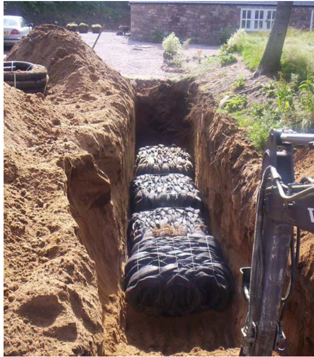
Figure 5.29 – Tyre bale soakaway construction, Highland, Summer 2005.
