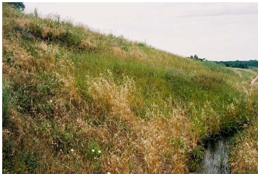
Figure 5.13 – Water drained to the front of the slope by layers one and two of the tyre bales around two years after the completion of construction.
