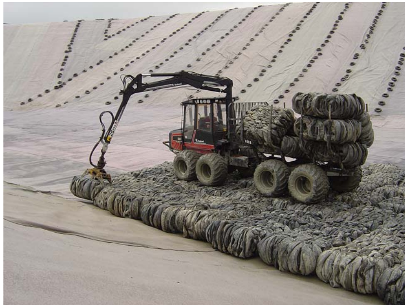
Figure 6.4 – Use of a ‘loggers’-clam’ to handle tyre bales.
