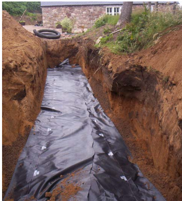
Figure 5.30 – Tyre bale soakaway construction, Highland, Summer 2005.
