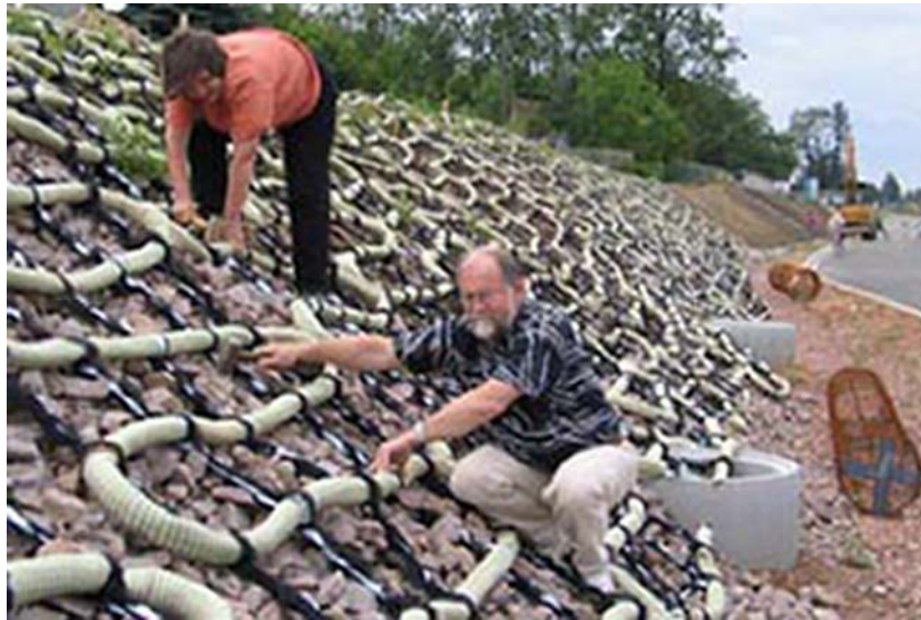
Figure 6.10 - Anti-erosion 'rope' geogrid for the promotion of vegetation growth on steep slopes developed by the Saxon Textile research Institute in Chemnitz, Germany ( http://www.tu-chemnitz.de/tu/presse/artikel/forschung1.php?aid=114 ).
