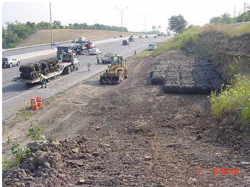
Figure 5.11 - Placing the second layer of tyre bales in the excavated IH30 slope failure, the covered first layer can be seen below the tyre bales in the picture. (Photograph © Texas Department of Transportation.)
