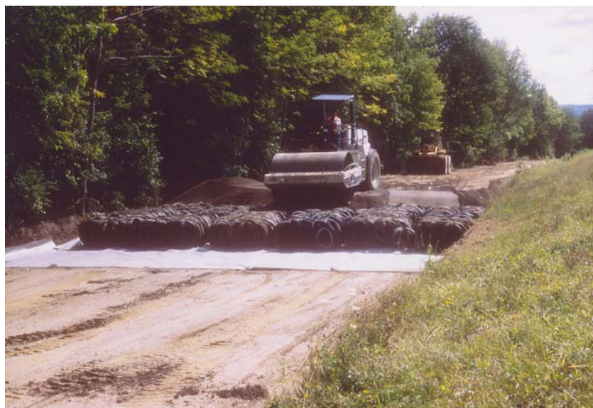
Figure 5.4 – Vibrating material between the bales and compacting the layer above the bales. (Photograph © Chautauqua County Department of Public Facilities.)
