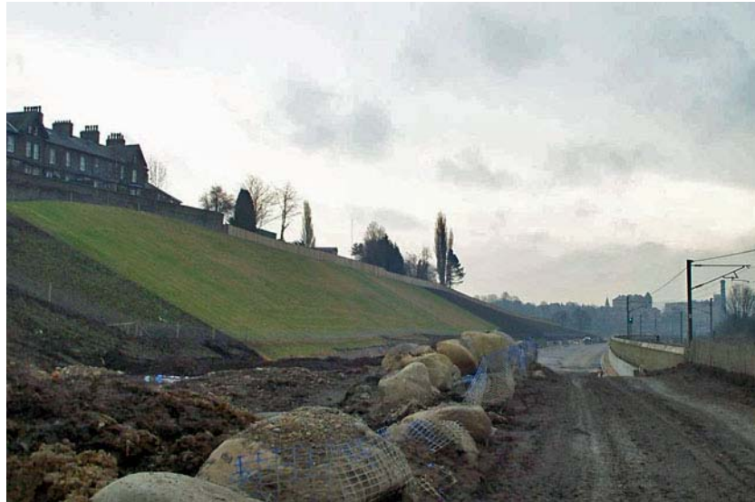
Figure 6.8 – Slope successfully constructed at 1:1.9 on the A650 Bingley Bypass (from Osborne, 2005, with permission).
