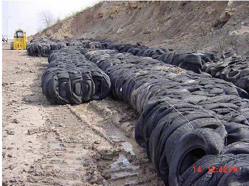
Figure 5.10 – Placing the first layer of tyre bales in the excavated IH30 slope failure. (Photograph © Texas Department of Transportation.)
