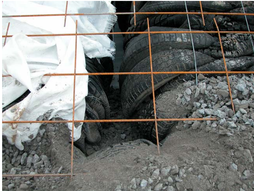
Figure 5.2 – Construction in which the bales have not been placed as close together as possible and in which the voids between the bales have not been well filled.
