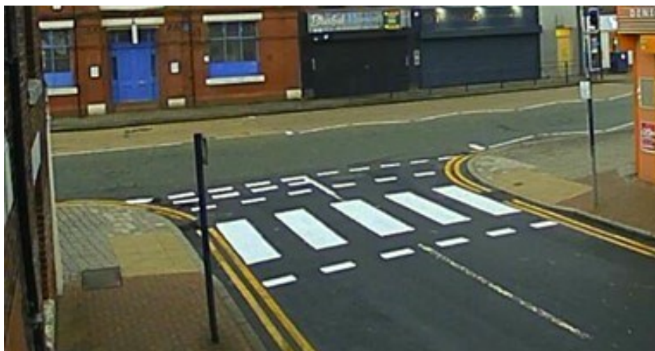
Figure 1: Example of a non-prescribed zebra crossing at one of the trial sites (from video)
