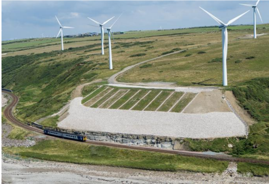
Figure 1: Regraded slope on the Cumbrian Coast Railway with Counterfort Drains. The upper slope above the rock fill blanket is clayey till and the area covered by the rock fill blanket is glacial sand (believed to be an esker). The counterforts also have slope (herring bone) drains to pick up localised water, they are generally concealed by the rock fill blanket. This highlights the need for detailed as built records to aid with future inspections, analysis and maintenance. Note the crest drain for the slope outfalls via a reno mattress lined channel on the right-hand side of the (image J. Murphy and Sons Ltd.)
