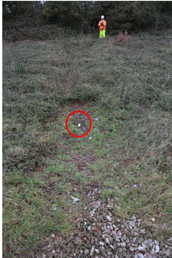
Figure 7: Settlement of drainage media at the junction with a feeder drain, in this case a herringbone drain. A 13cm scale can be seen towards the top-centre of the image within the red circle (A30, SGM 2065, January 2021)
