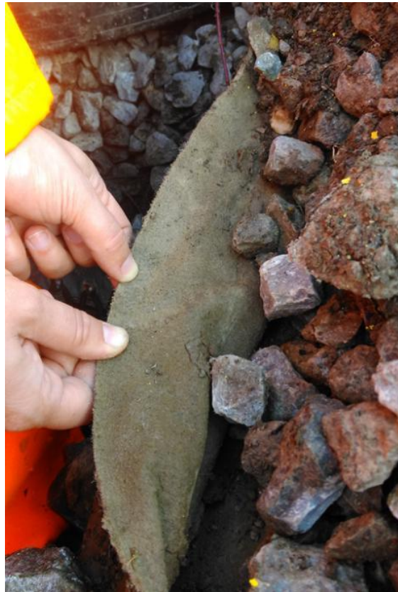
Figure 21: Geotextile filter separator on the upstream edge of a filter drain which had become fouled with fines during construction. The filter drain contains Type B drainage aggregate which is also fouled by fines (image the authors)
