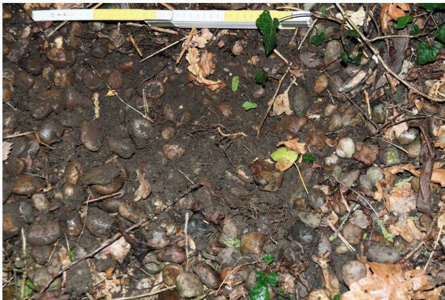
Figure 14: A counterfort drain that has become clogged over time with leaf litter, humous, fines and invasive roots (M42, SGM 9685, February 2022)
