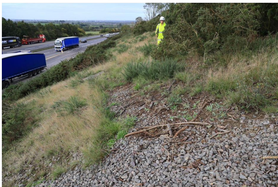
Figure 2: Vegetation debris from vegetation maintenance with the potential to block the structure of the drainage media (A14 [no SGM number, National Grid Reference NGR SP 62450 77600], October 2020)
