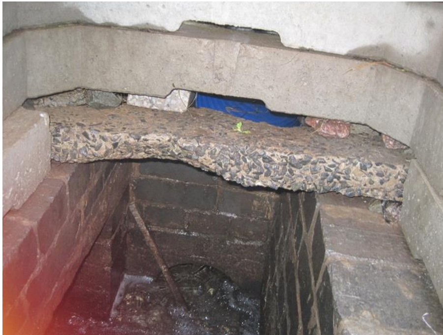
Figure 23: New upper level UPVC pipe (blue) installed above a historic clay pipe drainage system to increase the capacity of the drainage network. The upper pipe (blue) discharges against the sides of the catch pit rings as no opening has been formed (image the authors)
