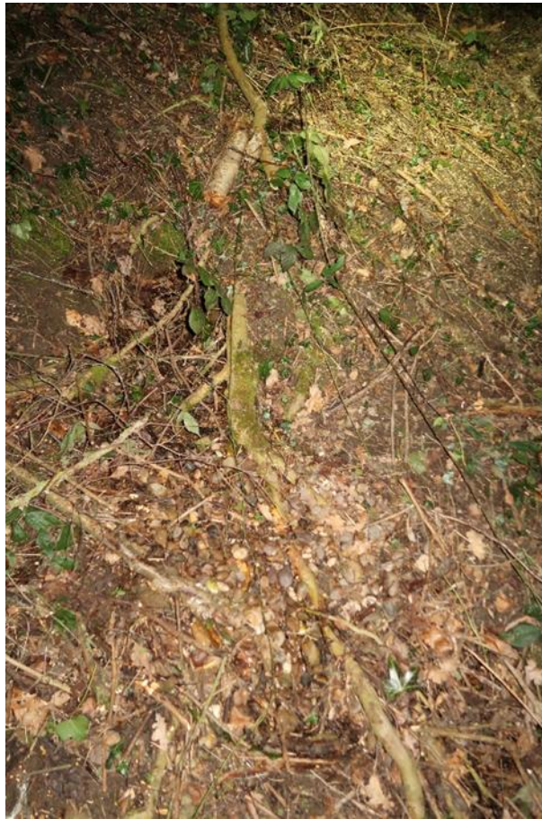
Figure 15: A counterfort drain with a series of tree roots following the drain (M42, SGM 9685, February 2022)
