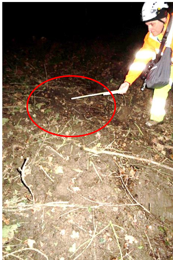
Figure 17: A spring-like feature at the head of a counterfort drain (M42, SGM 9685, February 2022)
