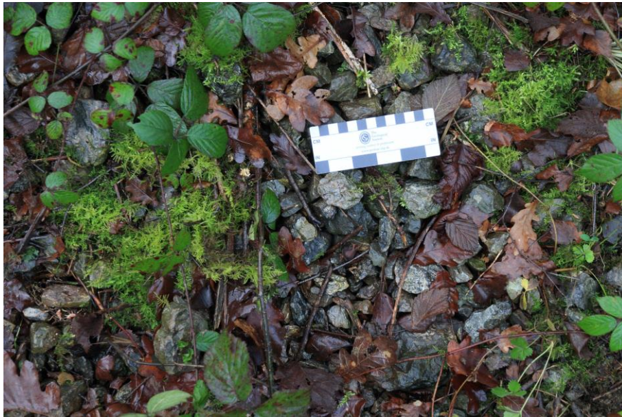
Figure 5: Vegetation debris and moss growing on the surface of a Counterfort Drain with the potential to clog the structure of the drainage media. (A30, SGM 1924, January 2021)
