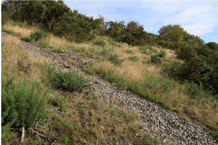
Figure 3: Vegetation debris from vegetation maintenance with the potential to block the structure of the drainage media (A14 [no SGM number, National Grid Reference NGR SP 62450 77600], October 2020)
