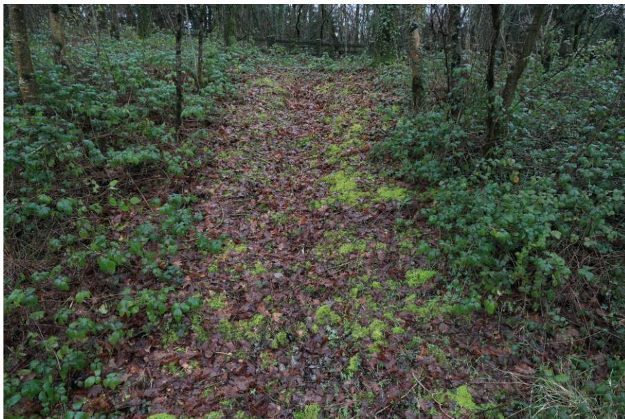
Figure 4: Vegetation debris with the potential to block the structure of the drainage media. The width of the drain is approximately 1.2m (A30, SGM 2053, January 2021)
