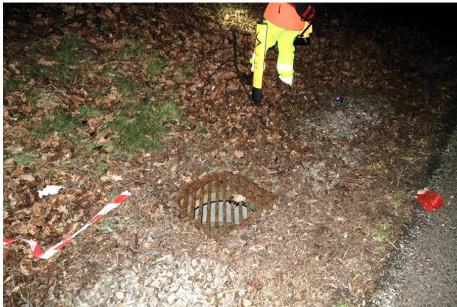
Figure 18: A vertical slope drain is located where the person is standing and the edge of carriageway filter drain runs along the verge with a grated catchpit visible in the foreground (M42, SGM 9685, February 2022)
