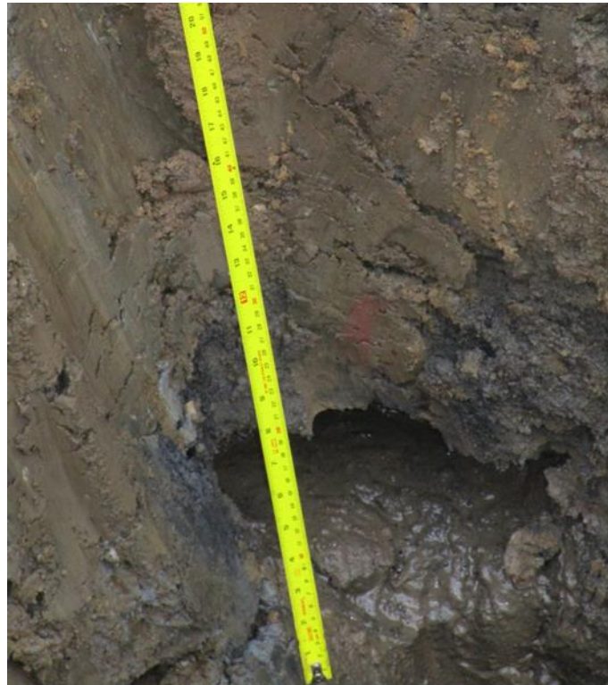
Figure 24: Example of a natural soil pipe, with significant water flow, encountered during the excavation of a crest drain above the location of a washout (debris flow) failure in till, west Cumbria (image the authors)
