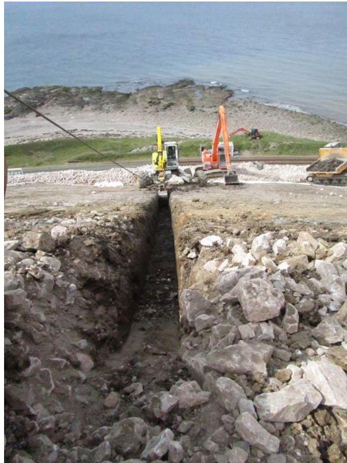
Figure 28: Tethered slope climbing excavator (Menzi Muck) installing Counterfort Drains on a large steep slope on the Cumbrian Coast Railway (image the authors: courtesy of J. Murphy & Sons Ltd)
