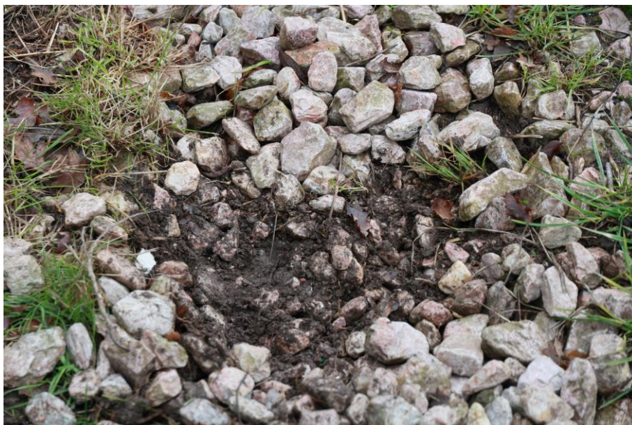
Figure 6: The effects rotted vegetation and soil migration into the drainage media can be seen by the degree of clogging in the centre of this approximately 1m wide Counterfort Drain; the aggregate sizes generally range from around 20mm to 90mm (A30, SGM 2065, January 2021)
