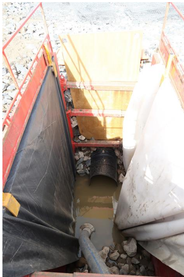
Figure 27: Filter drain excavation with trench support and over pumping of groundwater inflow on the Cumbrian Coast Railway (image the authors: courtesy of J. Murphy & Sons Ltd)
