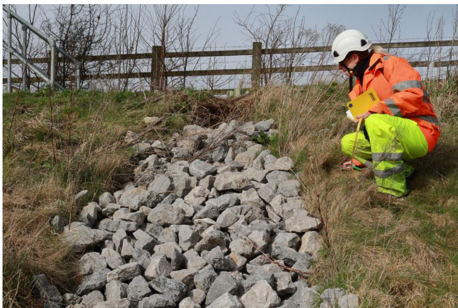
Figure 9: Settlement of large-sized drainage media at the head of a counterfort drain (M6 J34 northbound on-slip, no SGM number, NGR SD 49665 65240, March 2021)
