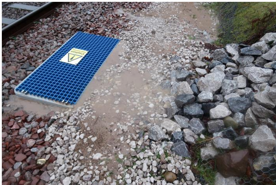
Figure 22: Toe of the Counterfort Drain in Figure 20 showing water issuing from the drain into the cess and carrying significant fines. The toe of the counterfort and the connection with the cess drain has become clogged by fines. Note that this is following removal of a previous build-up of deposited silt and sand (image the authors: courtesy of Network Rail)
