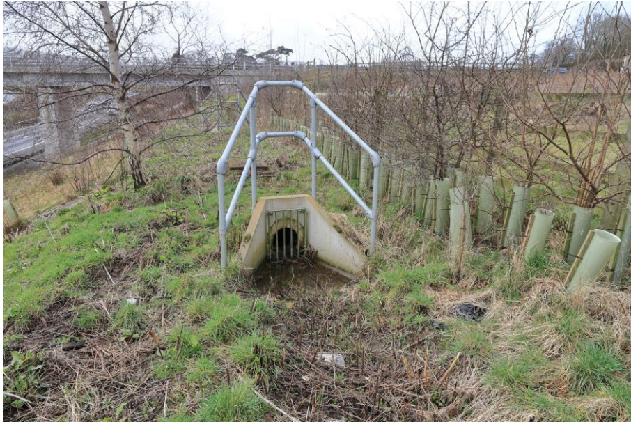
Figure 11: Slope crest drain and headwall intended to channel water into the counterfort drain below. Note the invert of the pipe is at a slightly higher elevation than the sidewall of the crest drain. As a result, water overtops the crest drain prior to entering the pipe and flows onto the slope and the Counterfort Drain below, see Figures 8 and 9 (M6 J34 northbound on-slip, no SGM number, NGR SD 49665 65240, March 2021)
