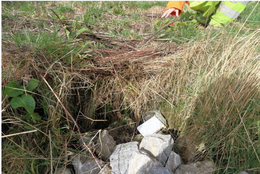
Figure 8: Settlement of large-sized drainage media at the head of a herringbone drain, that links to a counterfort drain (M6 J34 northbound on-slip, no SGM number, NGR SD 49665 65240, March 2021)
