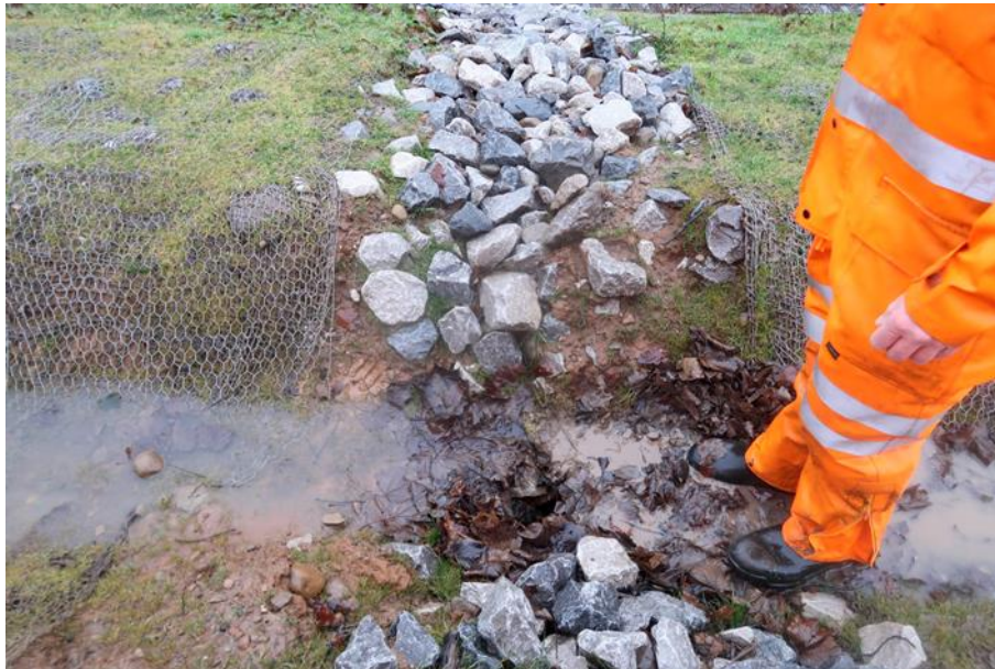
Figure 19: Direct connection of a Crest Drain into an un-modified Counterfort Drain. The rock fill (modified Class 6B) of the counterfort drain is exposed in the base of the Crest Drain. The rockfill has become clogged by leaf litter and soil carried by the surface water flow (image the authors: courtesy of Network Rail)
