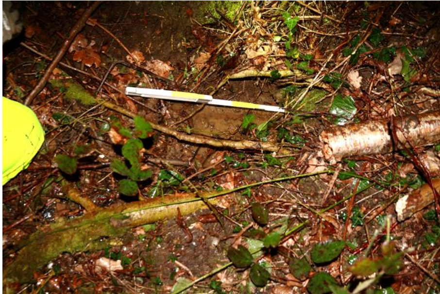
Figure 16: A spring like feature at the head of a counterfort drain (M42, SGM 9685, February 2022)
