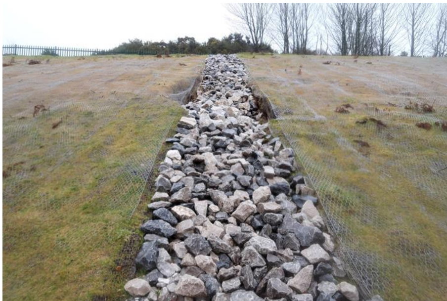
Figure 20: Collapse of a Counterfort Drain and surrounding slope due to internal erosion. The modified class 6B rockfill is in direct contact with the soils. Water could be heard flowing in the Counterfort Drain. The toe of the drain is shown in Figure 19 (image the authors: courtesy of Network Rail)
