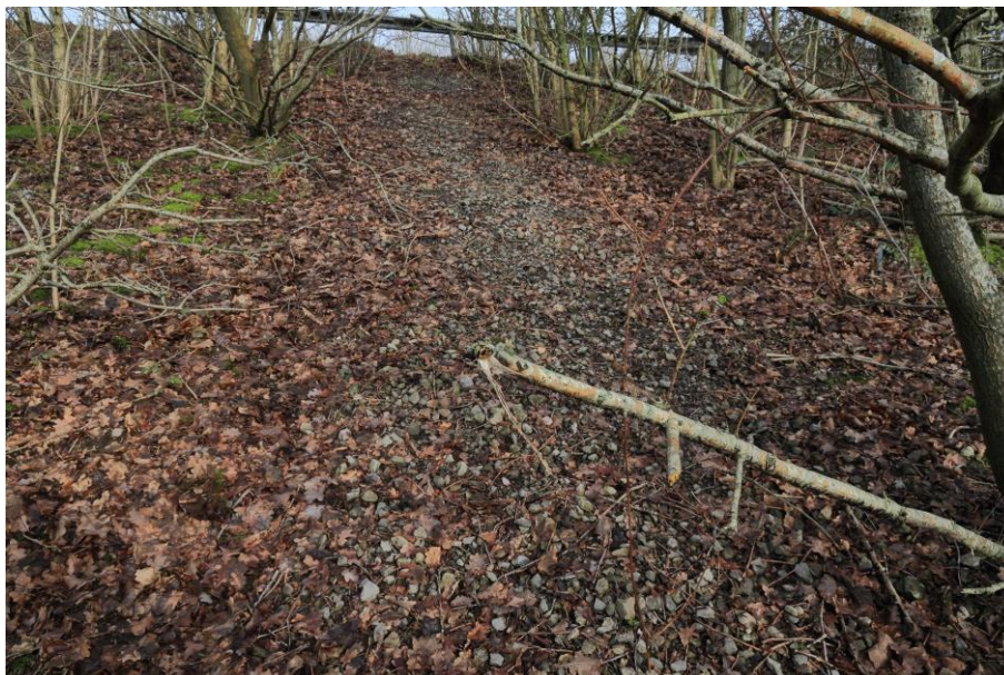
Figure 13: Counterfort constructed with the intention that it only act as a counterfort, that is without having a drainage function (A303, SGM 3329, January 2021)
