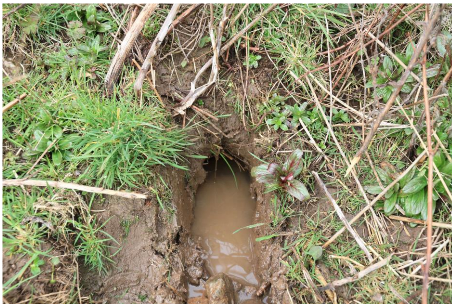
Figure 12: A land drain daylighting on the slope surface approximately 2m to 3m from the nearest counterfort drain (M6 J34 northbound on-slip, no SGM number, NGR SD 49665 65240, March 2021)
