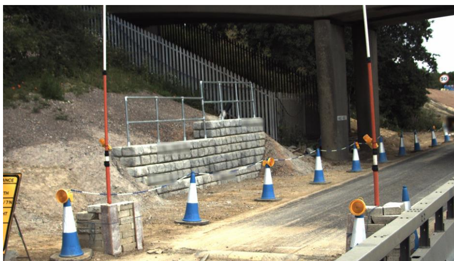
Figure 1: Modular Block Wall on M23 J9 (©AVIS)
