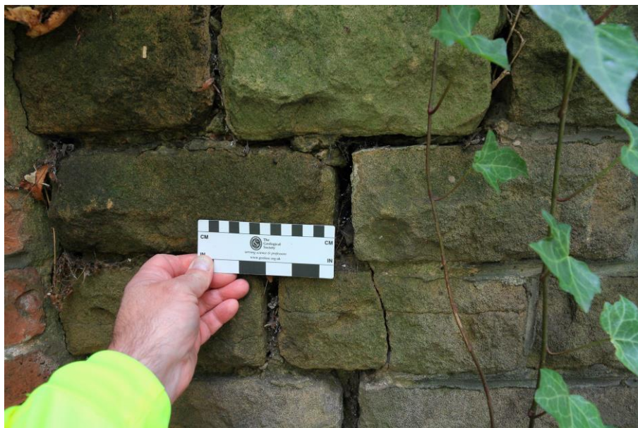
Figure 5: Cracking of stone block mortared wall (A52, SGM 9676, October 2020)
