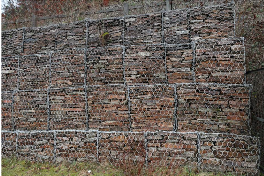
Figure 10: Gabion wall with local building stone used to provide an attractive front face (note that the use of the baskets at ninety degrees to their normal orientation is not considered to be problematic). These gabion baskets were the only instance of double corrosion protection observed during the site inspections. (A38, no SGM number, January 2021)
