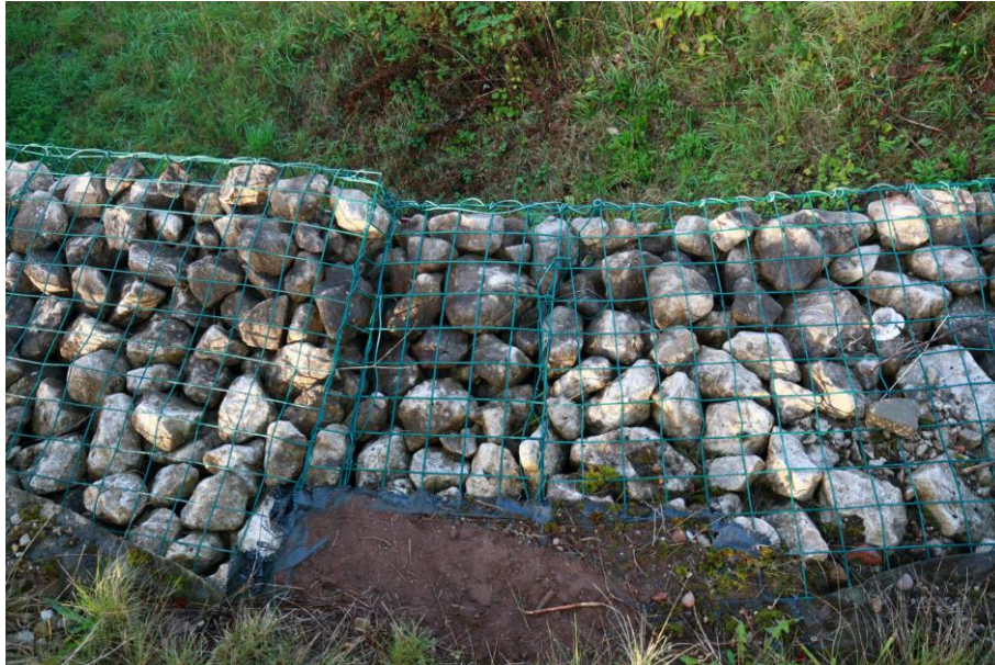
Figure 3: Top view of a curved Gabion Wall showing overlapping front panels (A38/A61 Junction, SGM 7630, October 2020)
