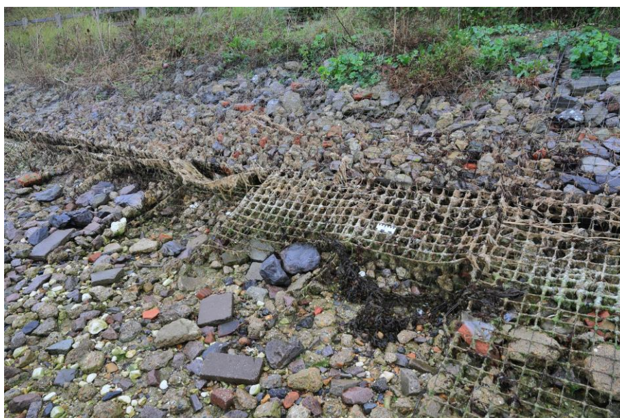
Figure 13: Gabions used within a marine environment leading to significant corrosion and loss of fill. The upper gabions are becoming undermined which will eventually lead to loss of support for the slope above (A27/M3 Junction, SGM 10797, October 2020)
