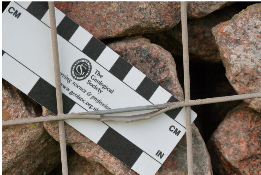
Figure 7: Coating peeling away from mesh on welded gabion basket (A453, SGM 4025, October 2020)
