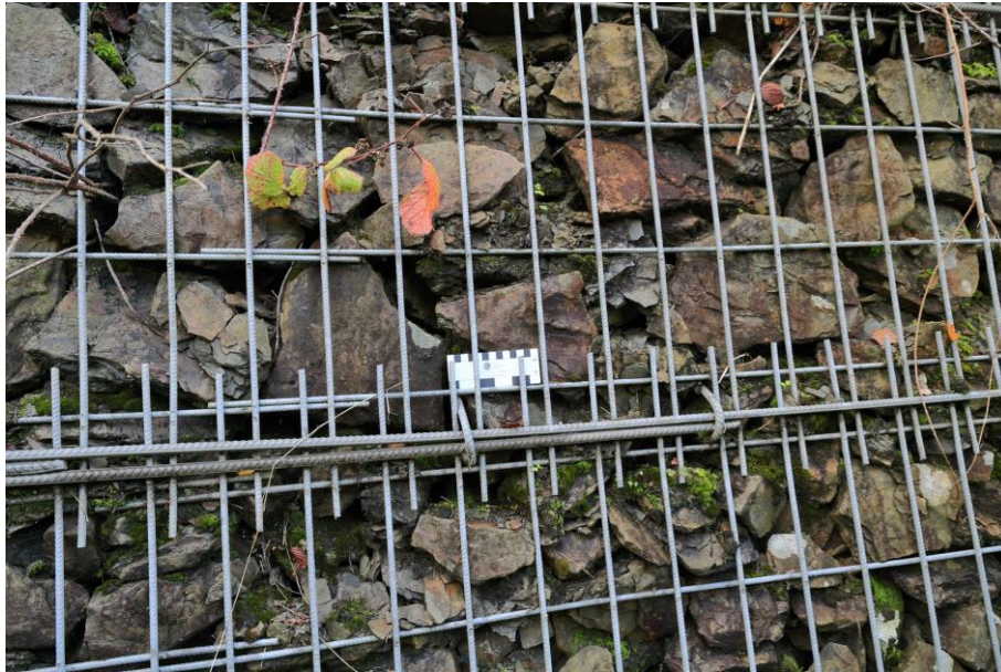
Figure 8: Shale showing significant signs of deterioration: this material is considered not to meet the MCHW requirements (M60, SGM 7038, October 2020)
