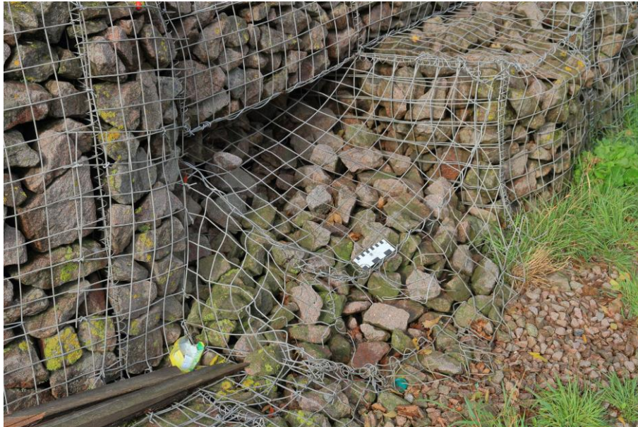
Figure 16: Helicoil springs used on the vertical edge joins of the welded mesh gabion baskets. Lower gabions struck and damaged by vehicle but upper baskets have remained in place despite the lack of support below (A453, SGM 4025, October 2020)
