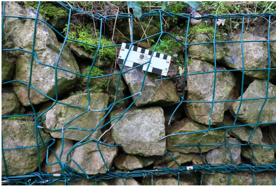
Figure 14: Vandalism of gabion basket which is located along a public footpath. The wire mesh appears to have been cut (A45/A46 Junction, SGM 9117, October 2020)
