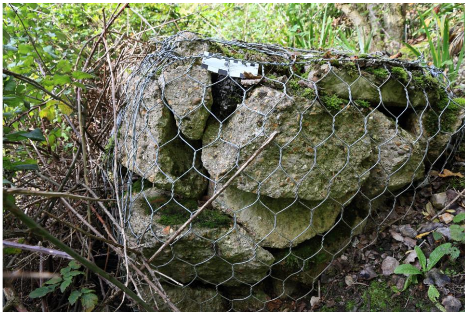
Figure 9: Oversize concrete fill leading to large voids within the gabion baskets. The oversize fill also means that the gabions have been unable to be properly sealed along the top, instead they are secured at pinch points where the fill allows (A42, SGM 6082, October 2020)
