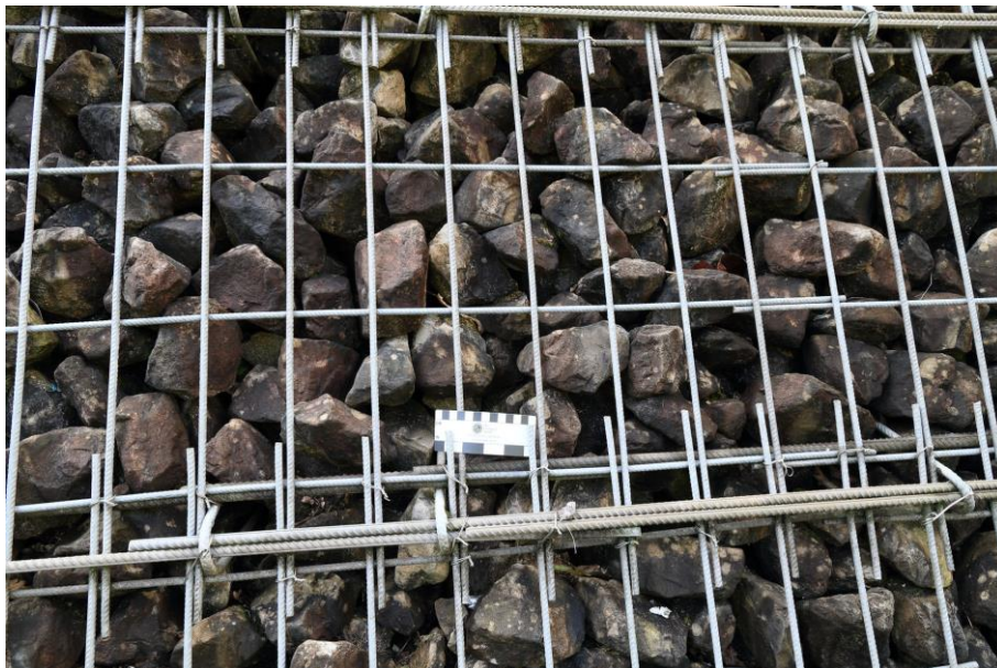
Figure 11: Gabion-type wall with a significant proportion of undersized material that could be readily removed from behind the mesh by hand (M60, SGM 7066, October 2020)
