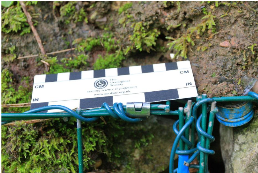
Figure 5: Plastic coating peeling away at the edges of the gabion basket where the mesh and wires have been cut (A45/A46 Junction, SGM 9117, October 2020)
