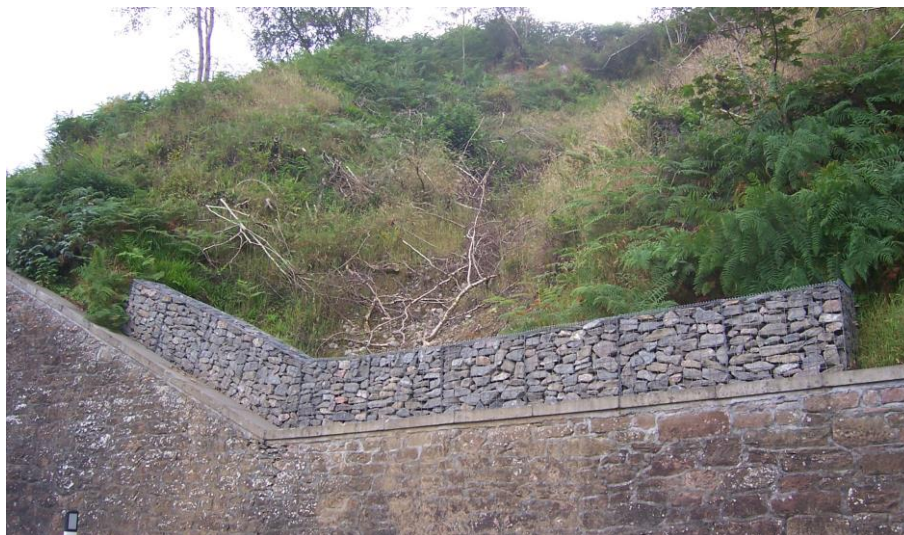
Figure 1: Example of a retaining structure formed from Gabion baskets (from Winter et al., 2009)
