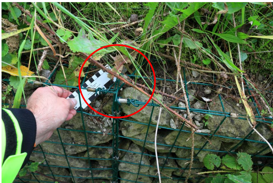
Figure 6: Top of gabion basket fastened to the adjacent basket compromising the structural integrity of the basket (M60, SGM 5281, October 2020)
