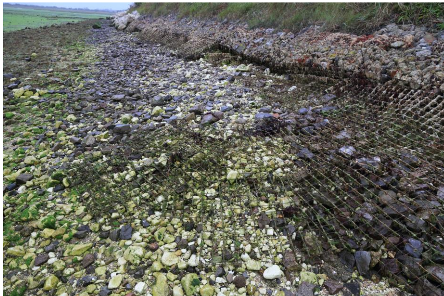
Figure 12: Gabions used within a marine environment leading to significant corrosion and loss of fill. The upper gabions are becoming undermined which will eventually lead to loss of support for the slope above (A27/M3 Junction, SGM 10797, October 2020)
