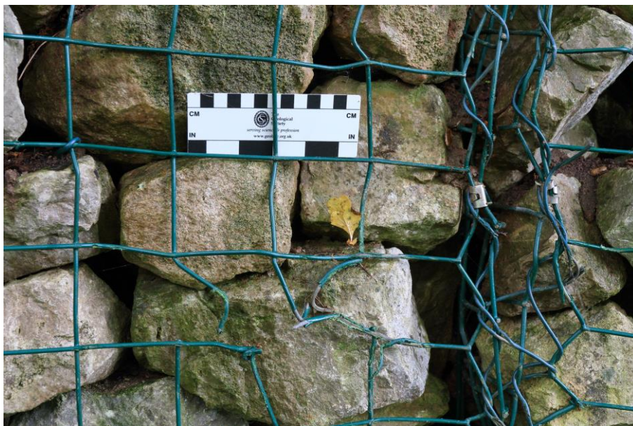
Figure 4: Large voids can be left if baskets that are not rectilinear are not filled correctly. The void reaches back for more than 0.5m behind the front facing stone in the left hand basket (A45/A46 Junction, SGM 9117, October 2020)
