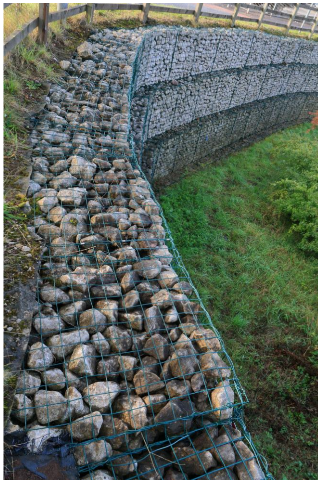
Figure 2: Curved Gabion Wall (A38/A61 Junction, SGM 7630 [unique SGM code from Atkins/Jacobs, 2020], October 2020)
