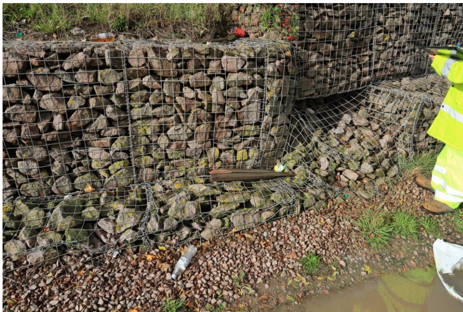
Figure 15: Vehicle overrun appears to be the primary cause of the significant damage to low height Gabion Wall at this location (A453, SGM 4025, October 2020)
