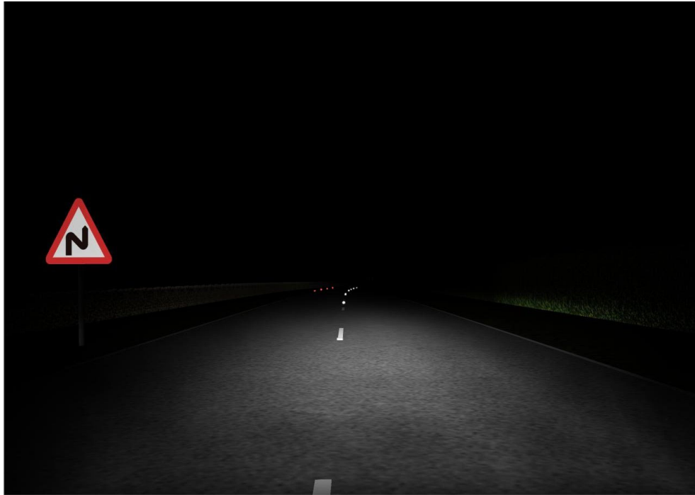
Figure C1. Picture 1 showed the road with Passive road studs in place.
