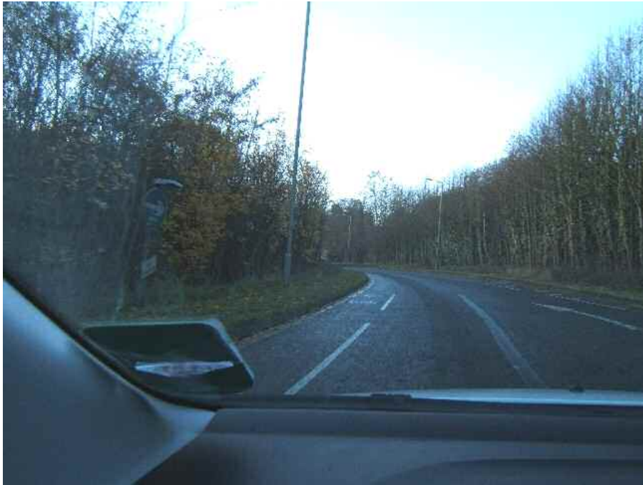
Figure 10: End of cycle path on A23 southbound.
