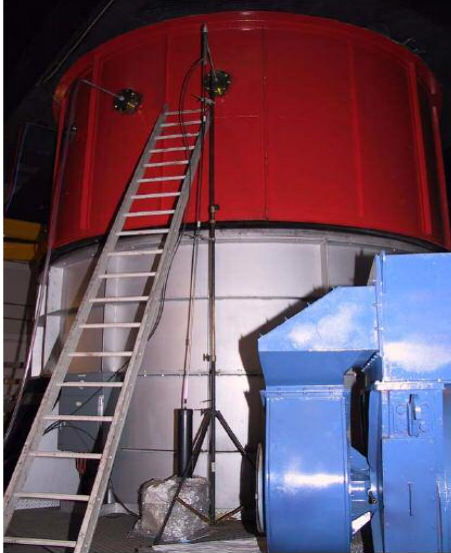
Figure B9-5: Promenade vent station – sampling through the fresh air shaft
