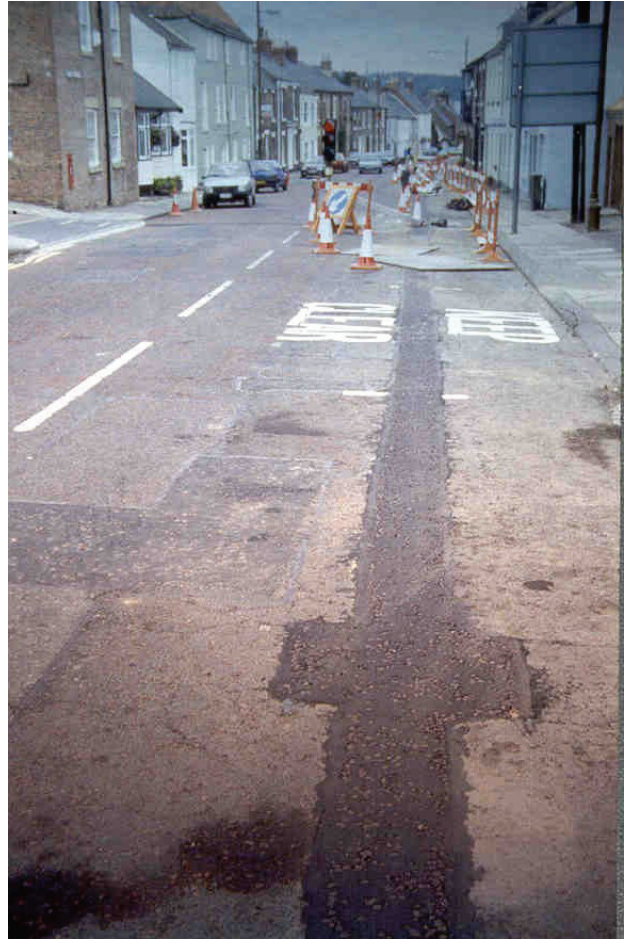
Figure 9 A carriageway with a longitudinal reinstatement
