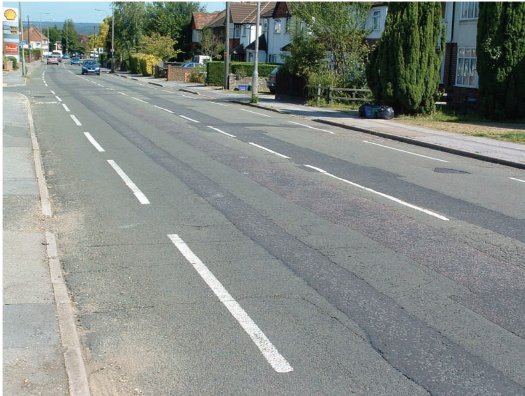
Figure 1 A heavily trenched carriageway
