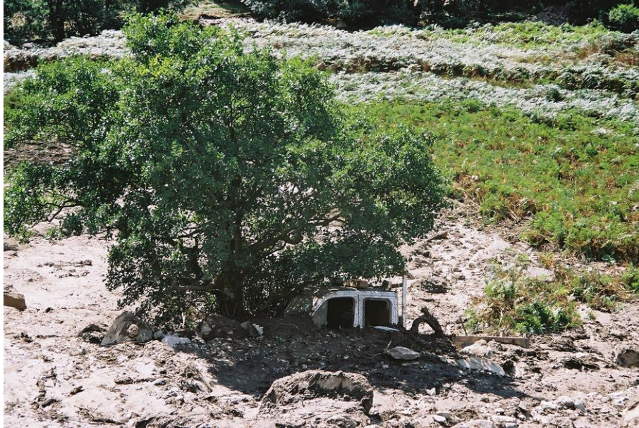
Figure 4. A85 Glen Ogle showing the Trunk Road Operating Company vehicle that was swept away by the northern debris flow. (From Winter et al., 2009.)
