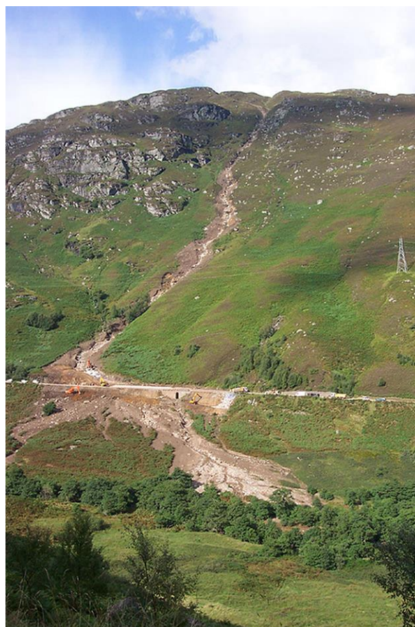
Figure 3. View of the northern A85 Glen Ogle debris flow two days after the event, showing the sharp bend in the channel just above road level. (From Winter et al., 2009.)
