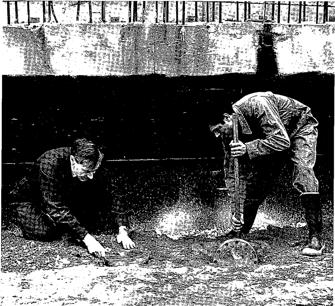
Plate 18 Installation of earth pressure cells
