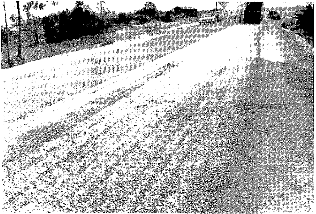
Fig.7.8 Longitudinal striations produced by a spray bar which is set too low.
