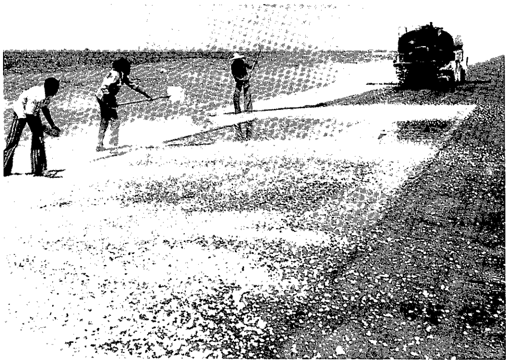
Fig.7.5 Surface dressing by hand.
