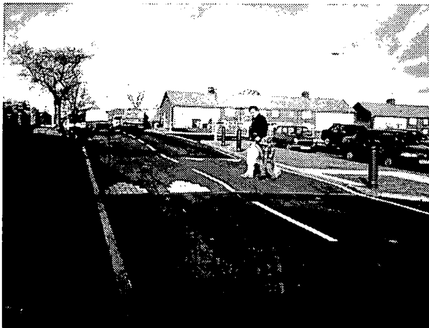
Fig. 9e Flat-top humps on Bushey Mill Lane outside no. 423
