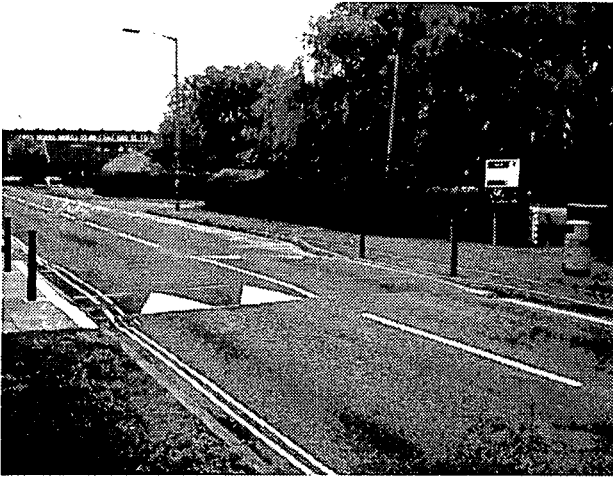
Fig. 4a Flat-top hump outside Mayfield County Junior School looking west along Mayfield Road
