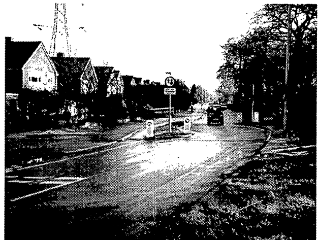
Fig. 9f Chicane on Bushey Mill Lane outside nos. 457/459, looking south
