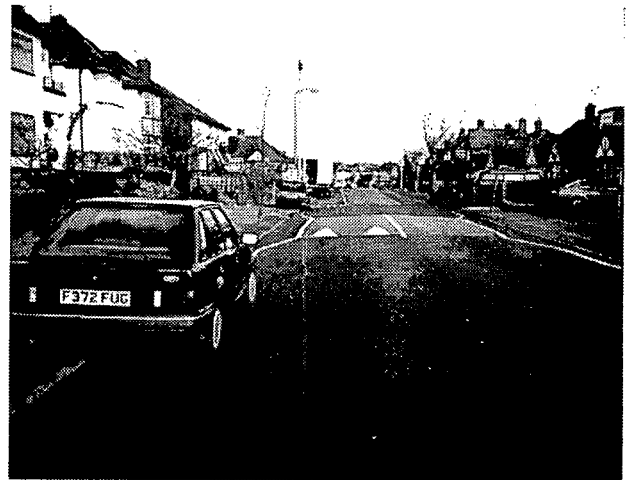
Fig. 9b Flat-top humps on Woodmere Avenue looking towards A41 (After)
