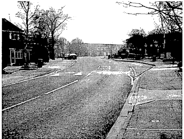
Fig. 7f Round-top humps on Ruddlesway looking southbound from location no. 6
