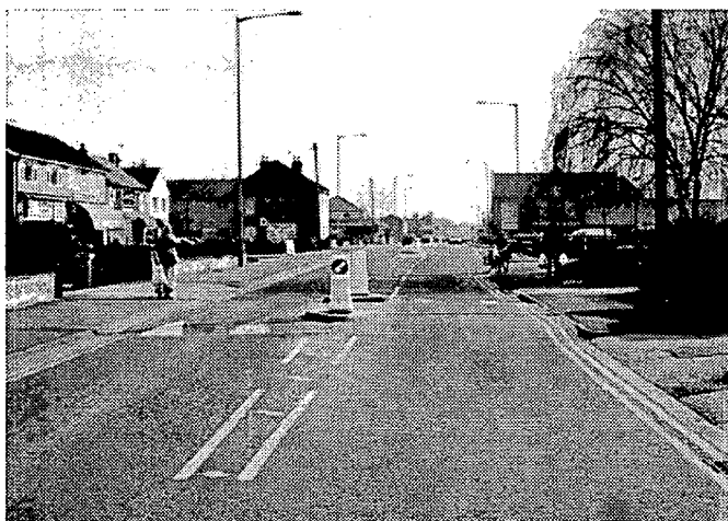
Flat-top humps and pedestrian refuges forming part of a distributor road traffic calming scheme at Dedworth Road in Windsor
