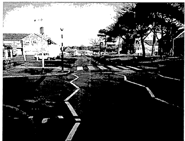
Fig. 9d Humped zebra crossing on The Gossamers outside no. 120
