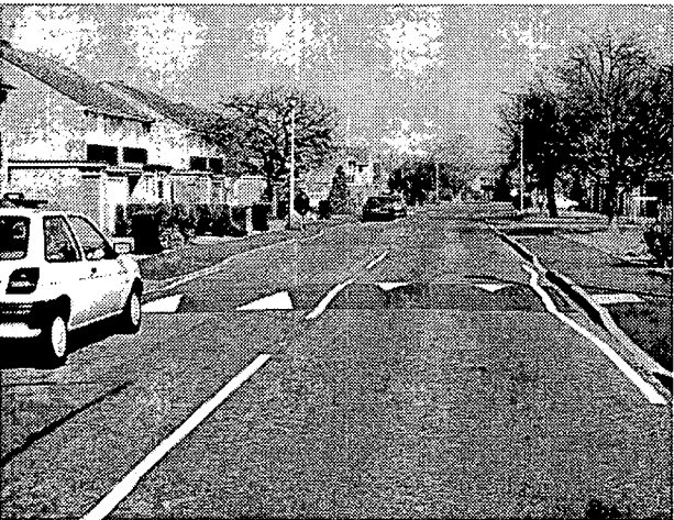
Fig. 7e Round-top humps on Gallys Road looking southbound from location no. 5
