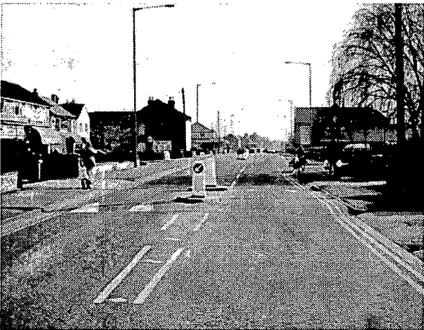
Fig. 7c Location no. 1 looking eastbound along Dedworth Road showing an 8.0 metre flat-top table with central island close to the new supermarket
