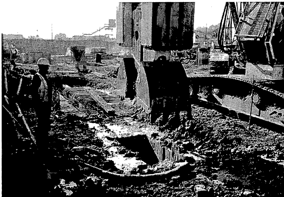
Fig 5. Excavation of the trench for a diaphragm panel
