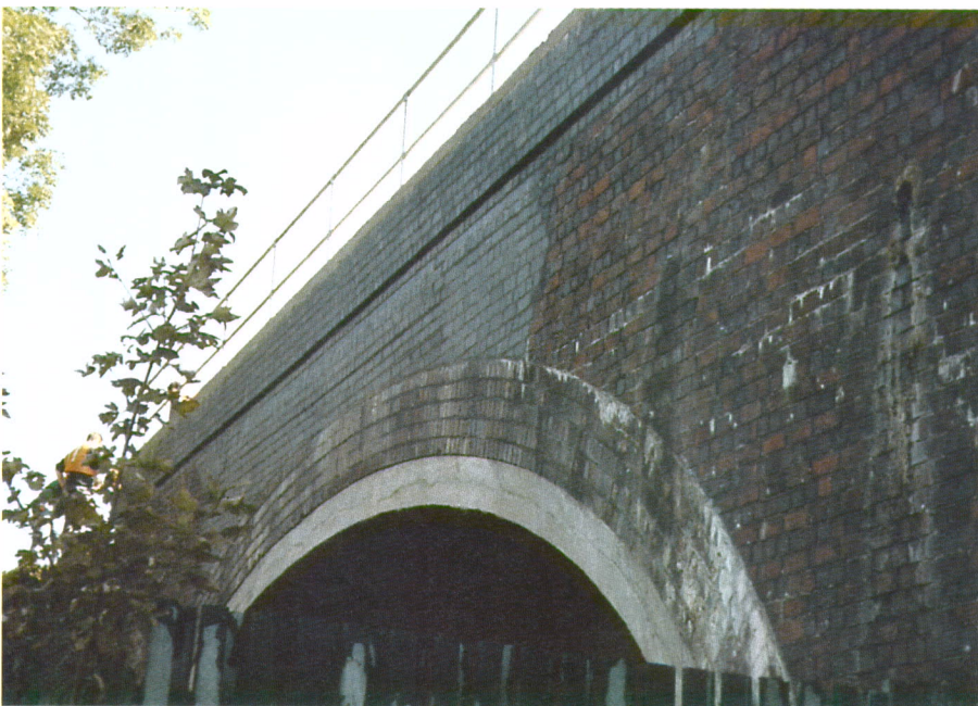
Fig.15 Sprayed concrete set in from edge of arch ring
