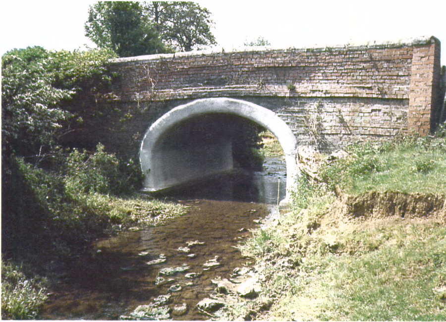
Fig.14 Sprayed concrete applied to face of arch ring
