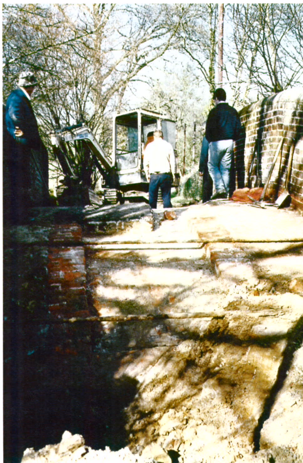
Figure 26. Poulters Bridge showing brick ribs on arch extrados
