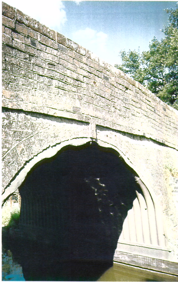
Fig.16 Corrugated liner applied to bridge with sloping spandrel wall
