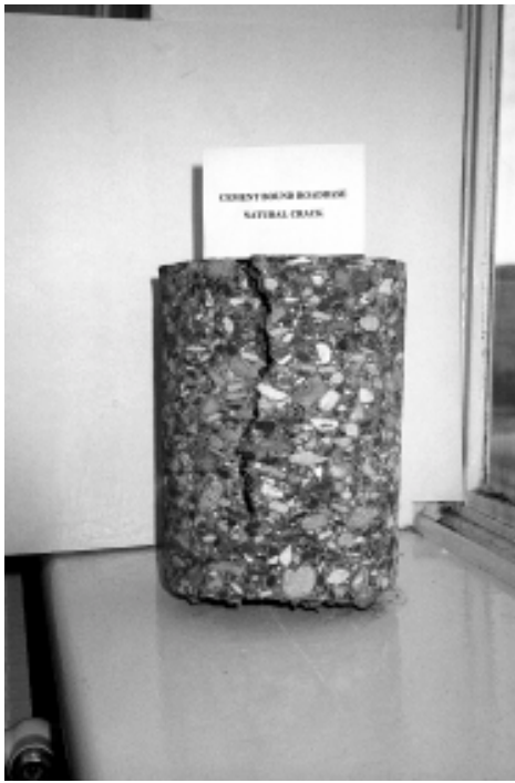
Plate 15 CBM core of natural crack
