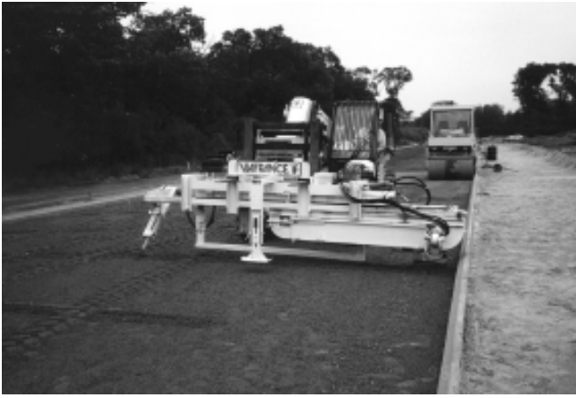
Plate 8 OLIVIA crack forming equipment
