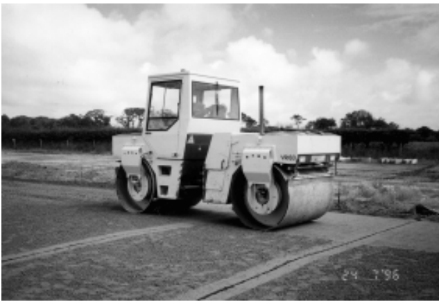
Plate 4 Compaction of vibrating plate induced cracks
