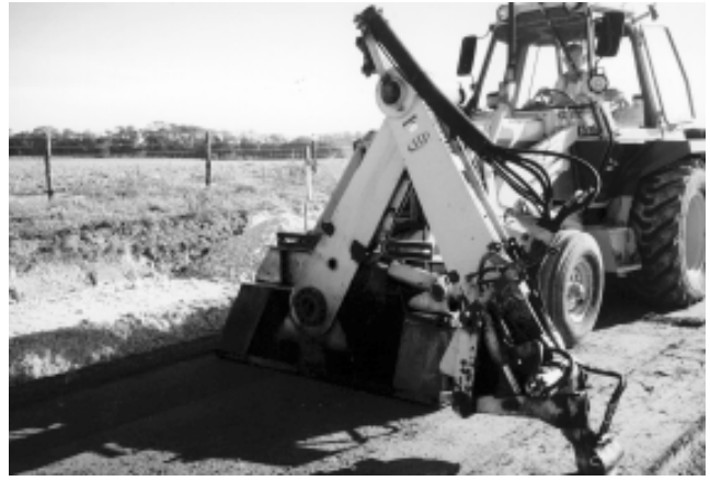
Plate 6 CRAFT pivot arm to traverse pavement layer
