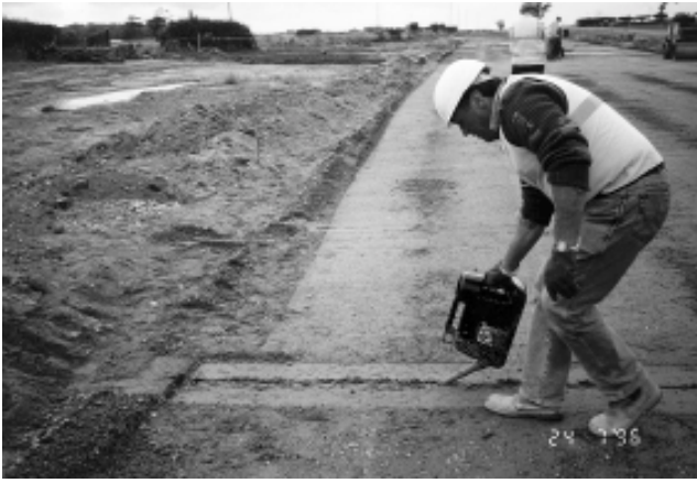
Plate 3 Inserting emulsion into vibrating plate crack
