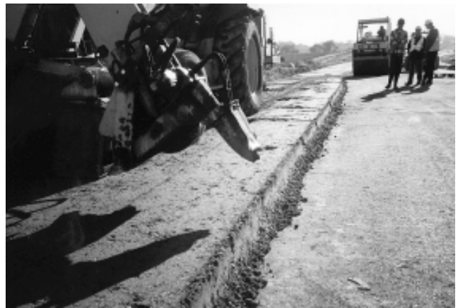
Plate 7 CRAFT crack forming blade
