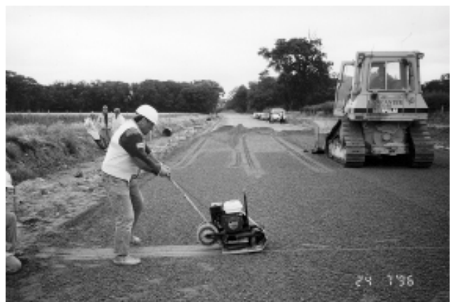
Plate 2 Vibrating plate traversing CBM roadbase
