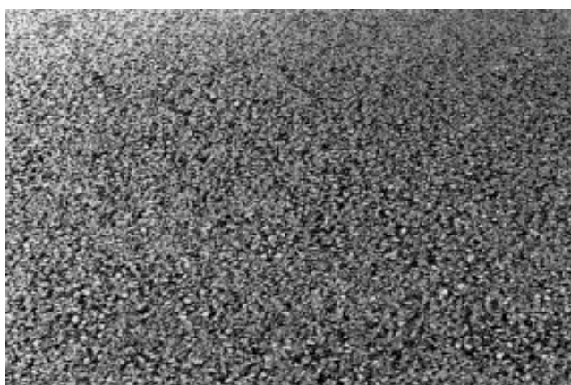
Figure 1 Texture of MILLOM HITEX after nearly 2 years on A635
