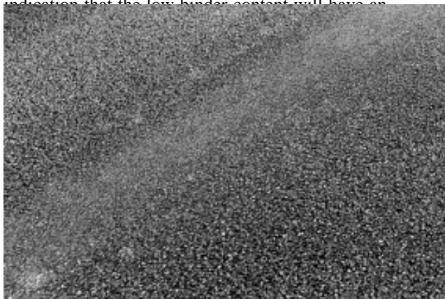
Figure 5 Difference in texture depth across lane of A635 after 2 years
