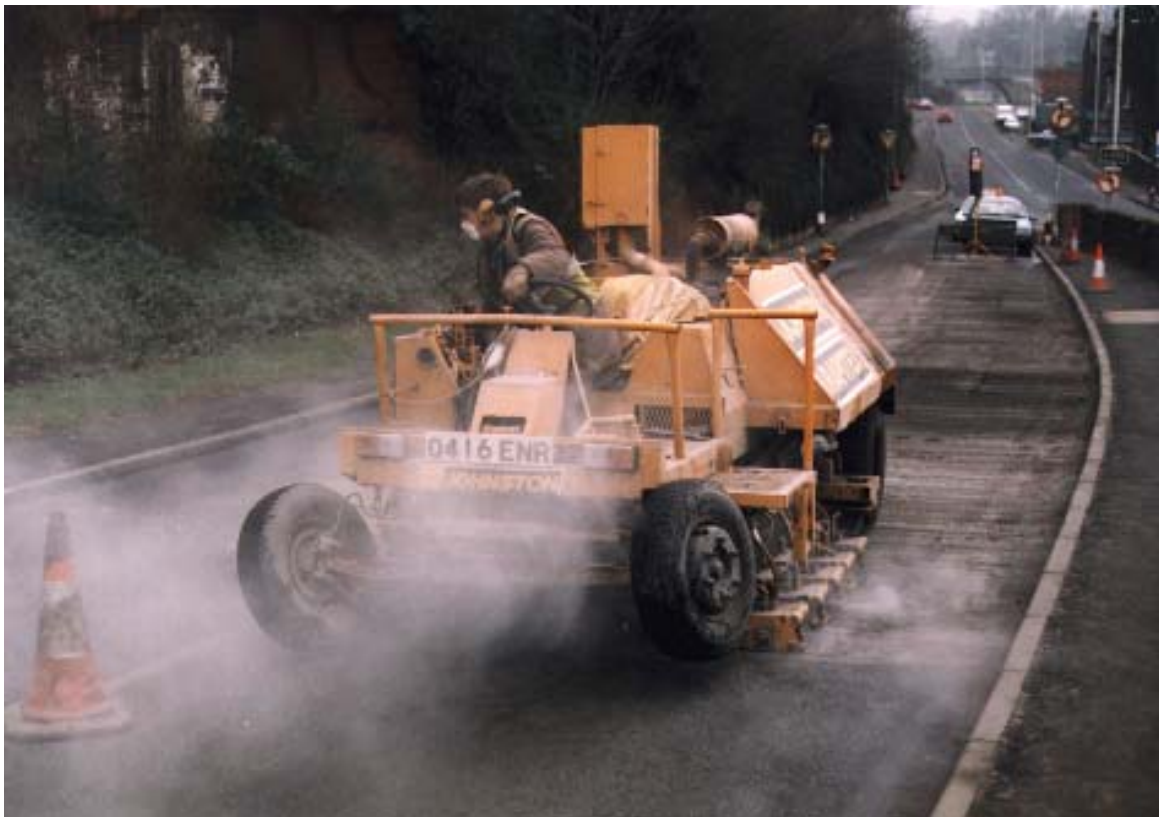
Photograph 20 Dust emissions from Rapitex Durogrip treatment
