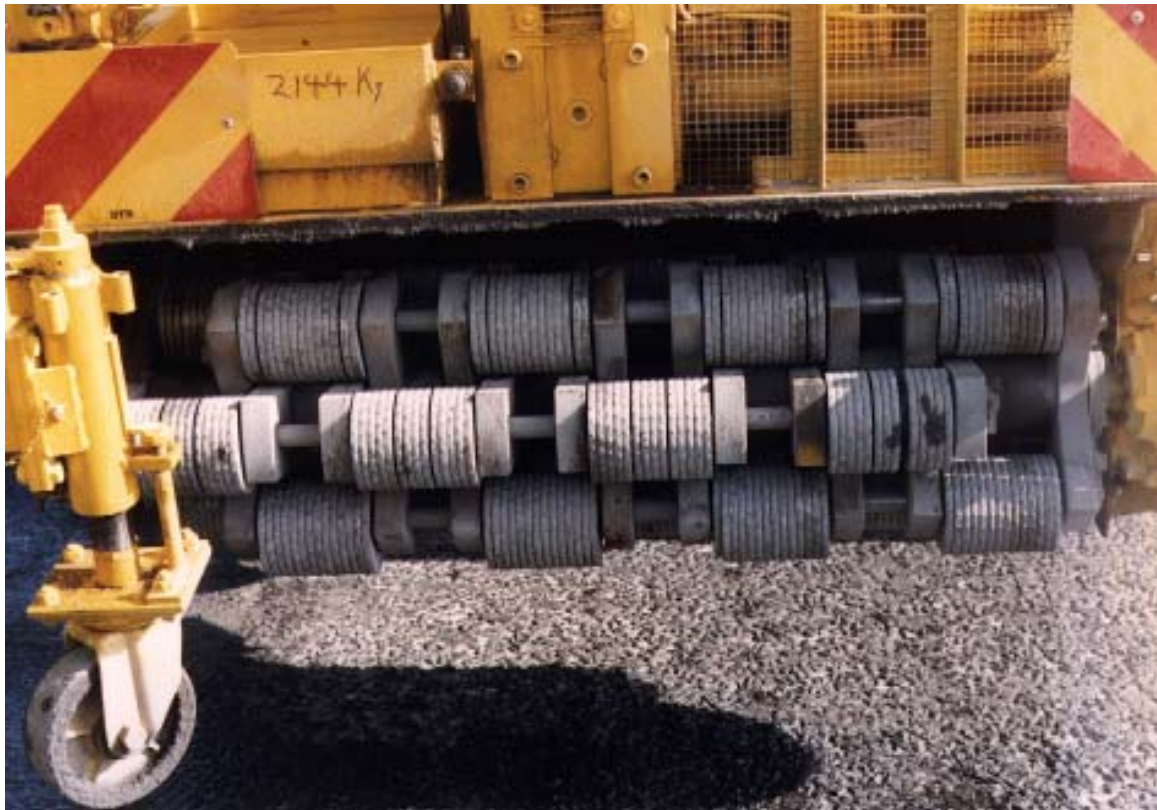
Photograph 9 Flail grooving cutters on Roadtex machine
