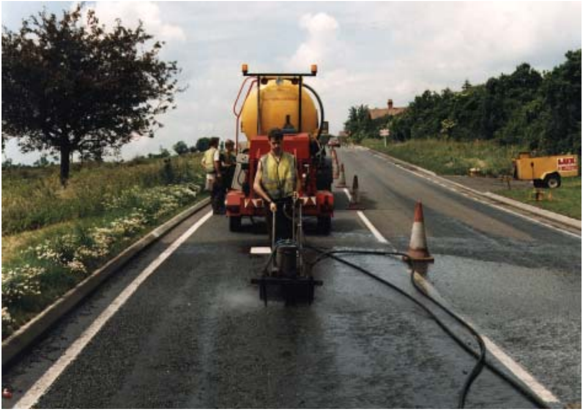
Photograph 17 Premier Road Treatment's Watertex machine
