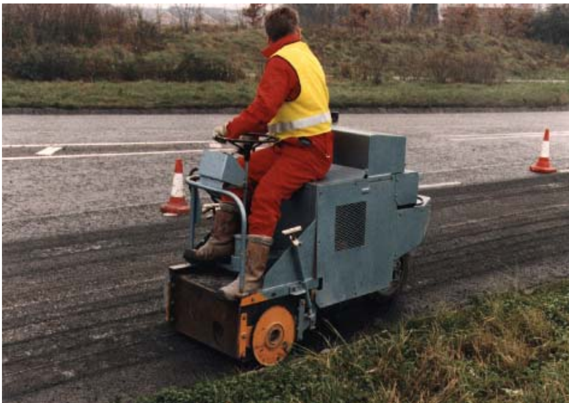
Photograph 12 Balvac Whitley Moran flail grooving machine
