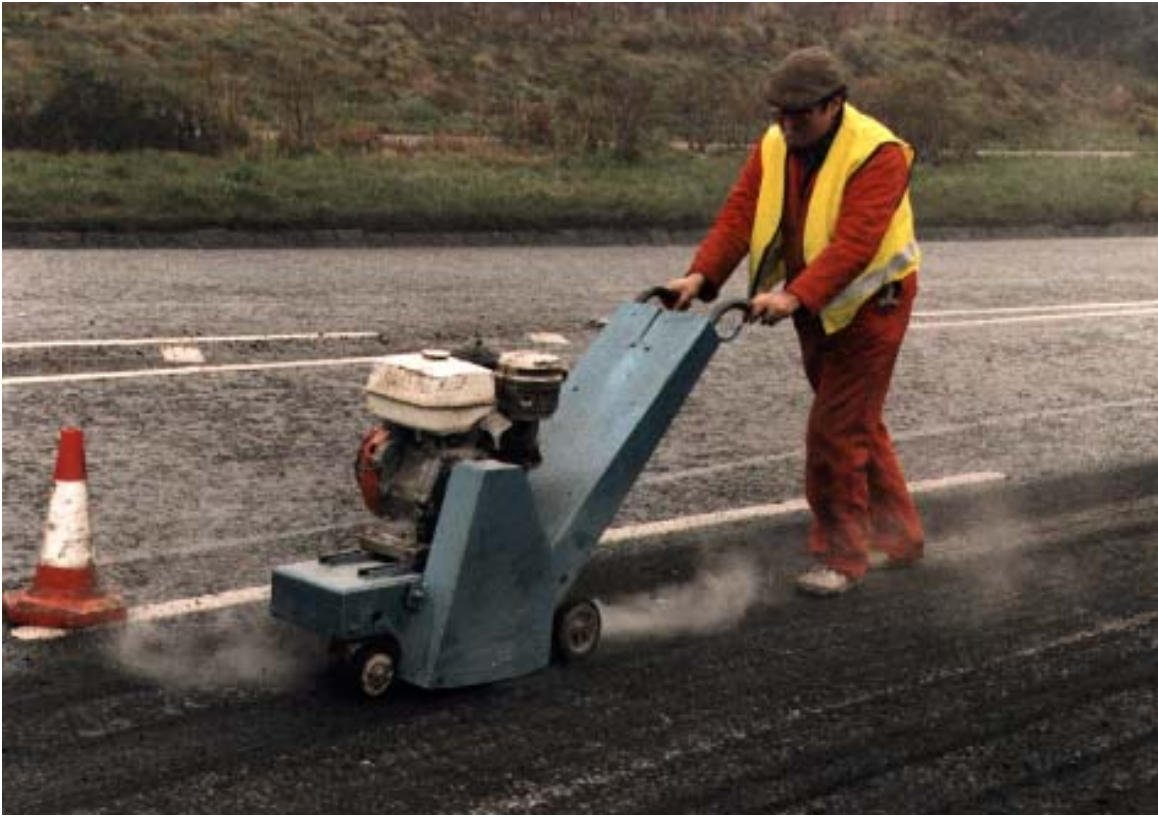
Photograph 21 Dust emissions from Balvac Whitley Moran treatment
