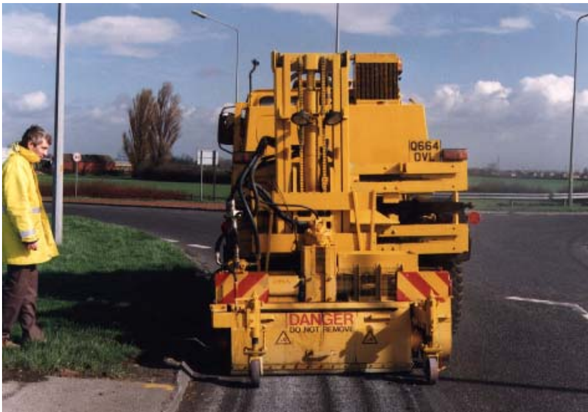
Photograph 8 Roadtex machine for flail grooving
