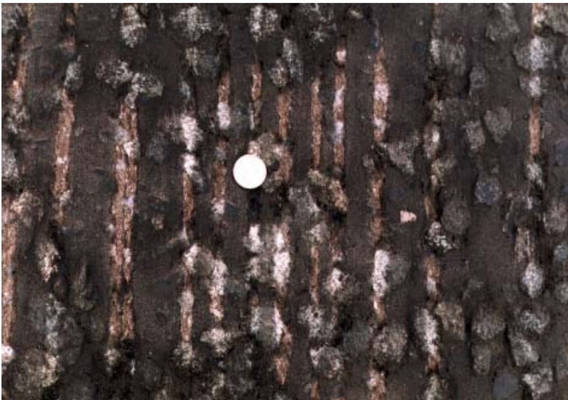
Photograph 10 HRA surface retextured by Roadtex
