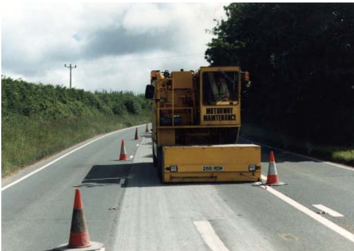
Photograph 1 Klaruwtex 190 bush hammering machine
