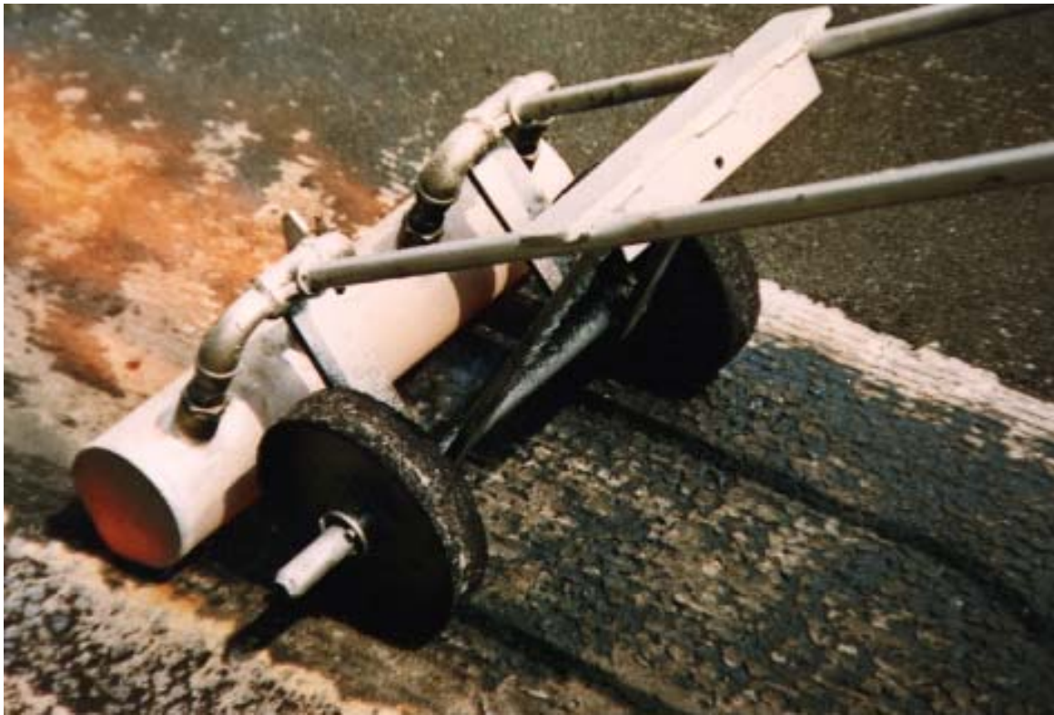
Photograph 11 Carbonising in conjunction with Roadtex treatment
