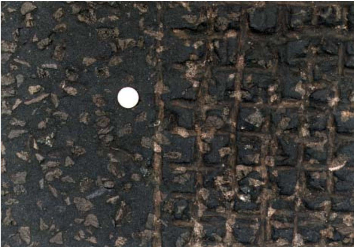
Photograph 16 HRA surface treated by Rapitex Durogrip process
