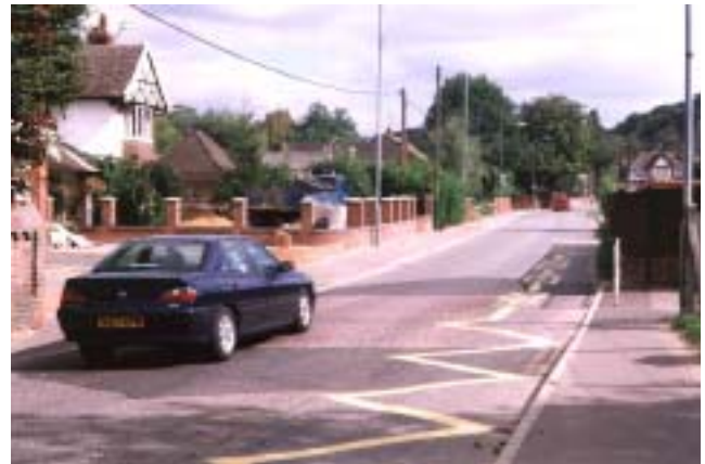
Figure 17 Flat-top hump, looking east
