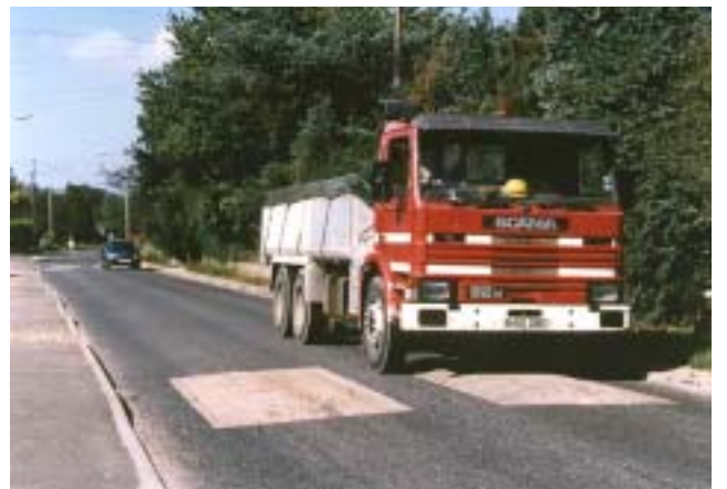
Figure 13 Car and HGV crossing speed cushion, West End
