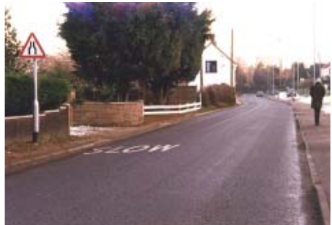
(d) West End (C171), looking east, about two-thirds of the way between junction with Longwater Lane and western entry to scheme. Speed cushions were installed along this stretch and related noise and radar speed measurements took place near the white cottage.
