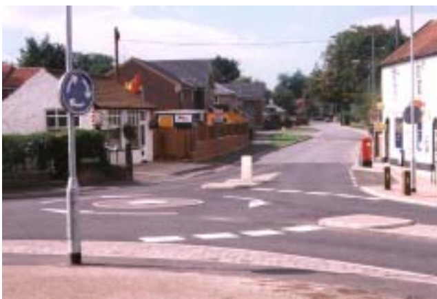
Figure 8 Mini-roundabout looking down West End where 20mph zone signing can be seen beyond the roundabout exit. The first pair of speed cushions can be seen beyond the signing. Block paved build-out with low kerb to permit overrunning in foreground; the roundabout island and refuge extensions show the same features
