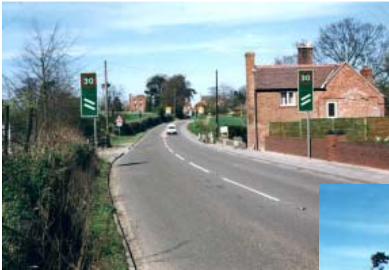
Countdown signs to the 30mph speed limit at the south gateway
