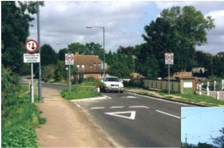
Southern entry to the 20mph zone, with a speed cushion within the narrowing (Longwater Lane)
