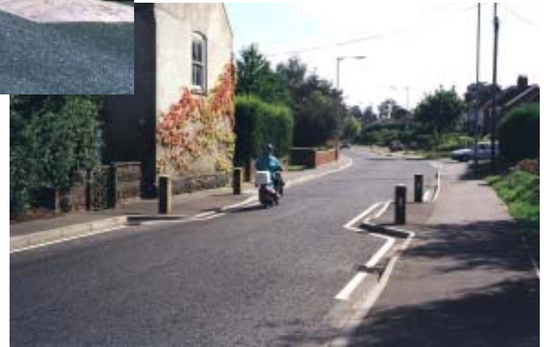
Single lane working narrowing (West End)
