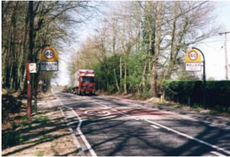
East gateway showing surface treatment intended to create the illusion of a flat-top hump (treatment repeated at intervals through village)
