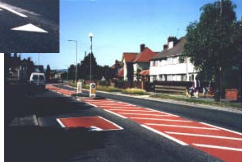
Speed cushion, pedestrian refuge and centre hatching just north of the village centre (looking north)
