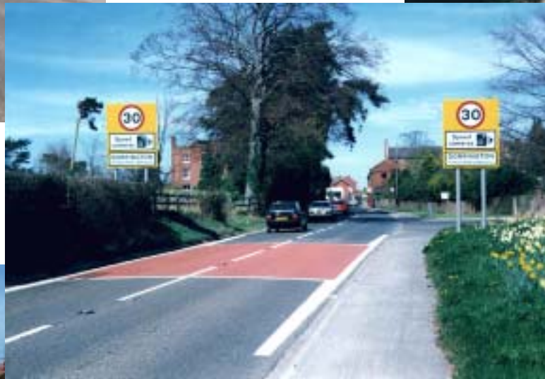
South gateway: red surface treatment and markings are repeated through the village
