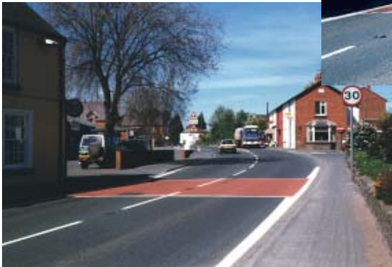
Repeated red patch with 30mph repeater signs in the village (looking north)
