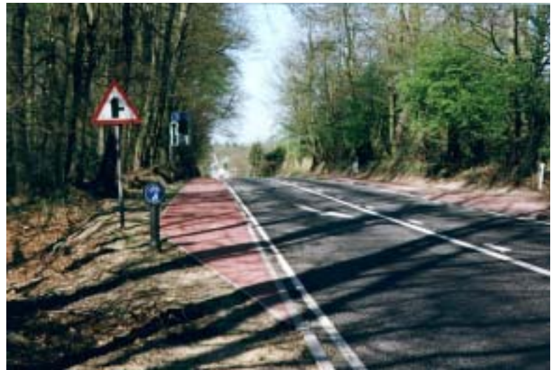
Start of footway converted to shared use by pedestrians and cyclists, just inside east gateway
