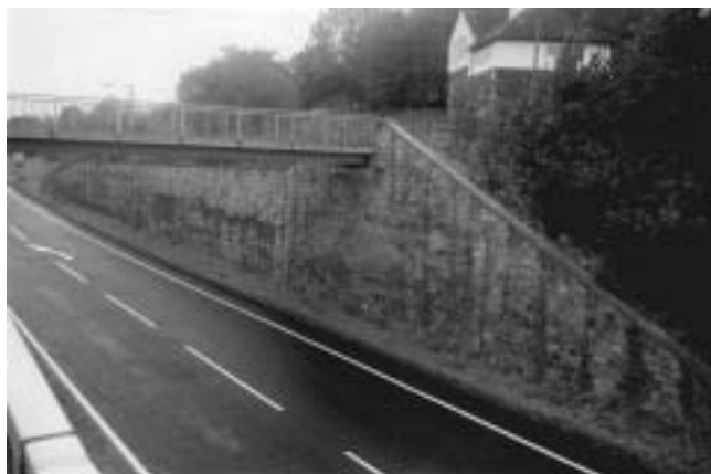
Figure 25 View of the anchored earth wall at Otley taken in October 1998
