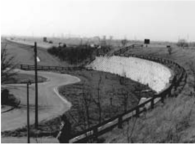
Figure 14 View of the completed reinforced soil wall at Whitley Bridge
