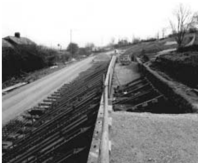
Figure 27 View of the construction works at the Otley site
