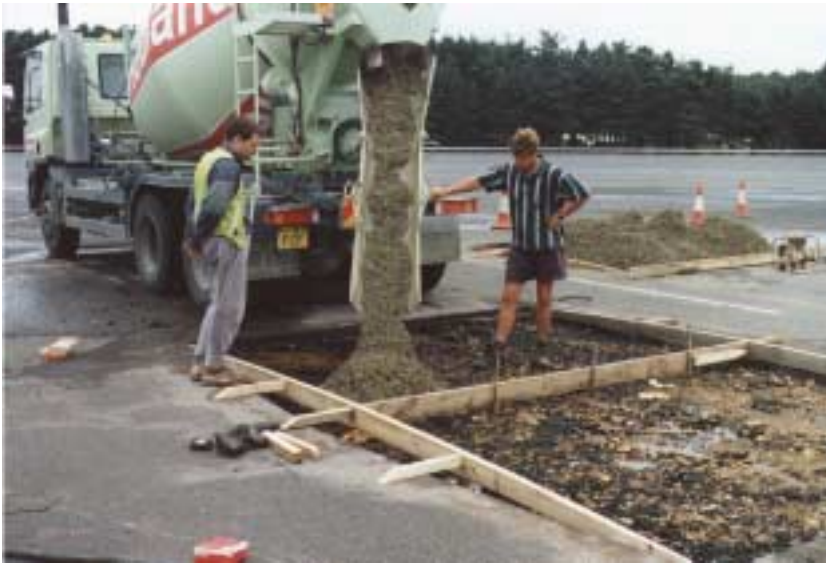
Plate 6 Construction of hump profiles, filling the formers with pre mixed concrete
