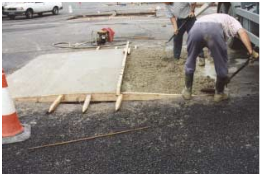
Plate 7 Construction of hump profiles, first half of hump compacted and leveled
