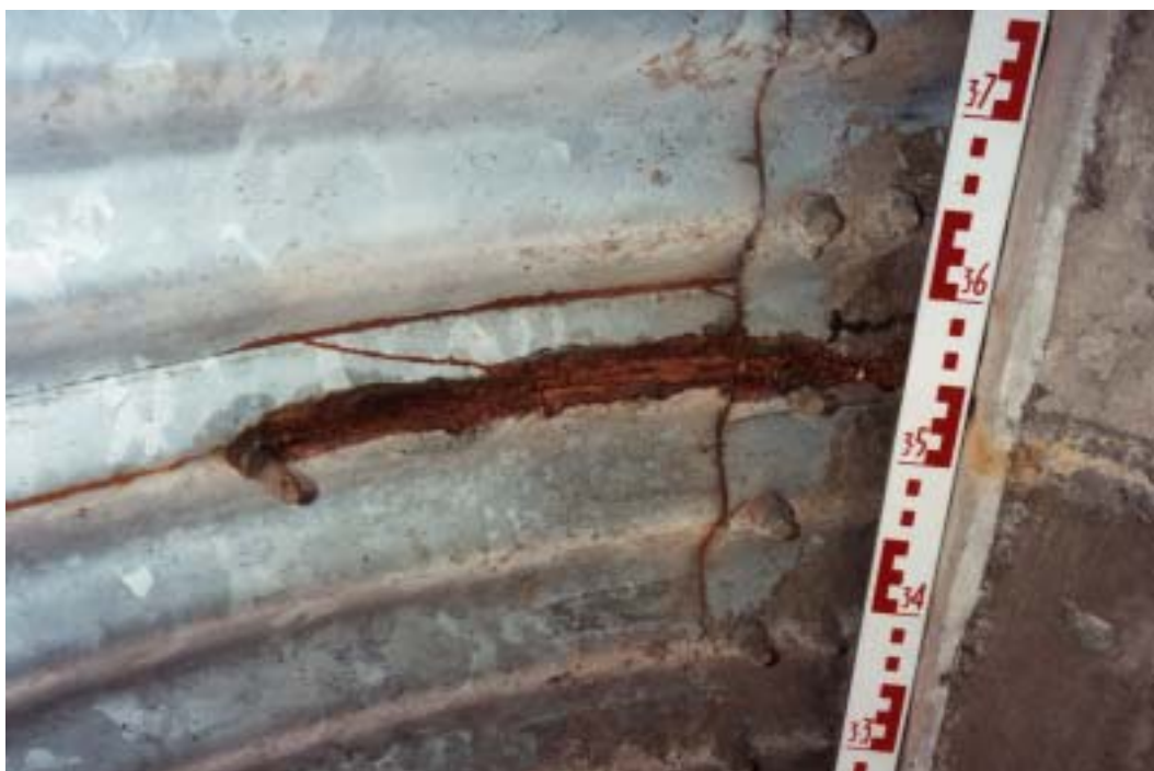
Plate 7.4 Corrosion to corrugated steel buried culvert on A564
