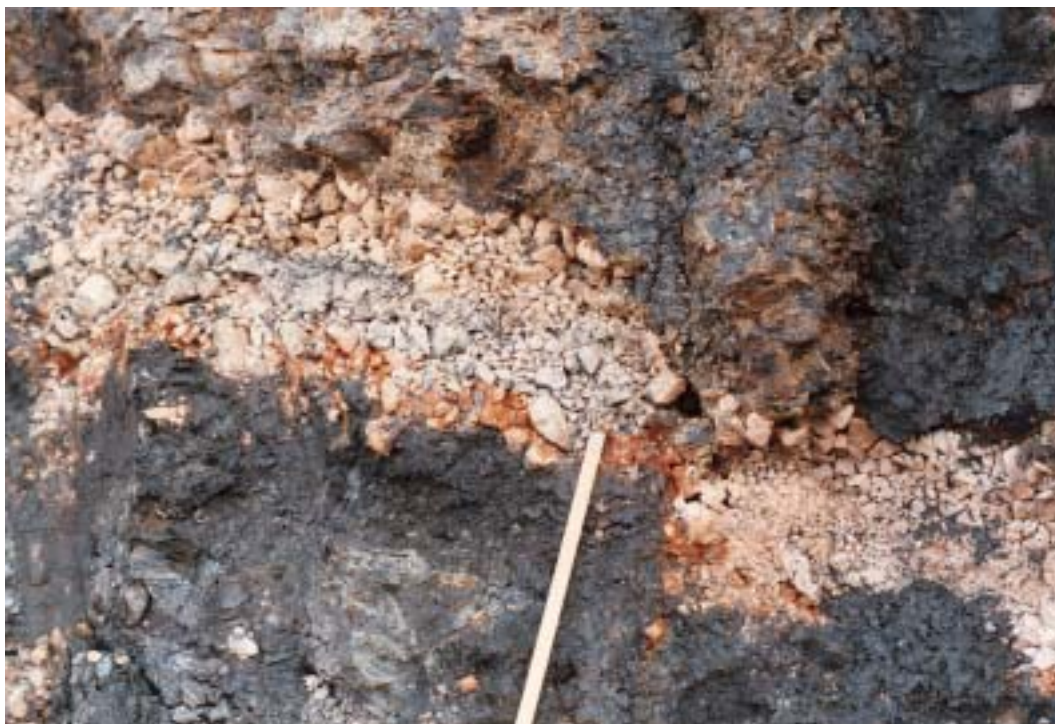
Plate 7.2 Chemical attack on limestone drainage blanket in acidic mudstone fill, Carsington Dam. Rupture surface to right of tape measure
