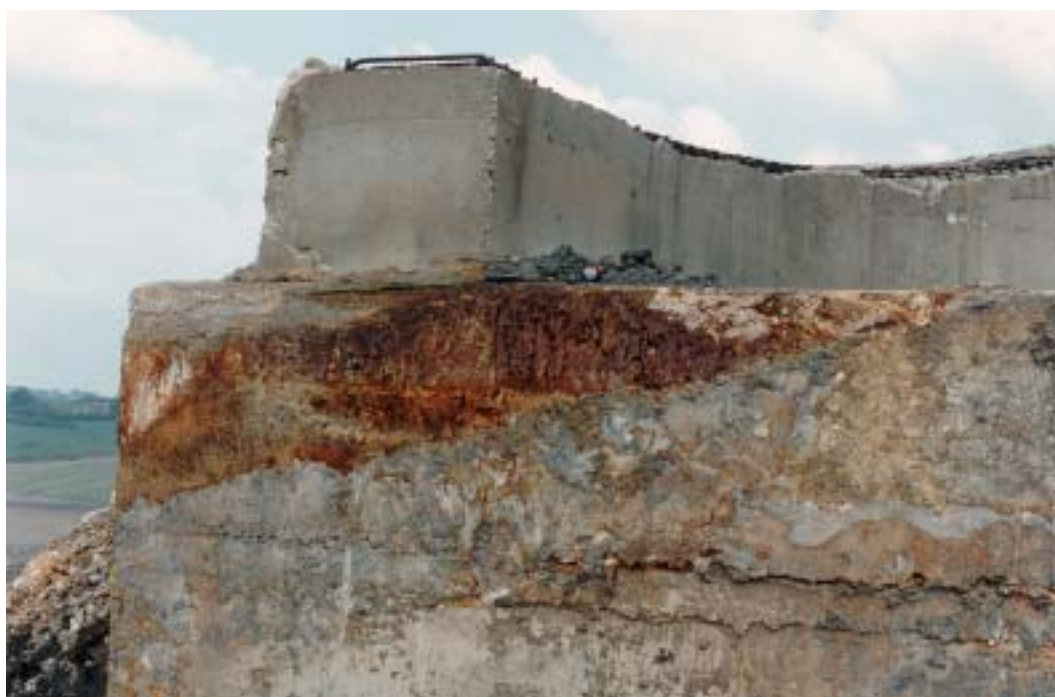
Plate 7.1 Concrete corrosion on spillway, Carsington Dam
