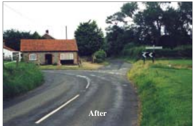
Figure 29 Wiveton: Village green, looking north along C599 (bending left) towards The Street (going ahead). Direction signing replaced by finger post arrangement; one chevron reduced in size and the other replaced by wooden marker posts
