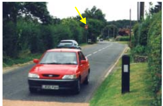
Figure 17b Fibre-optic 30 miles/h reminder sign (arrowed) just inside west gateway, being triggered by car approaching it (looking towards village)
