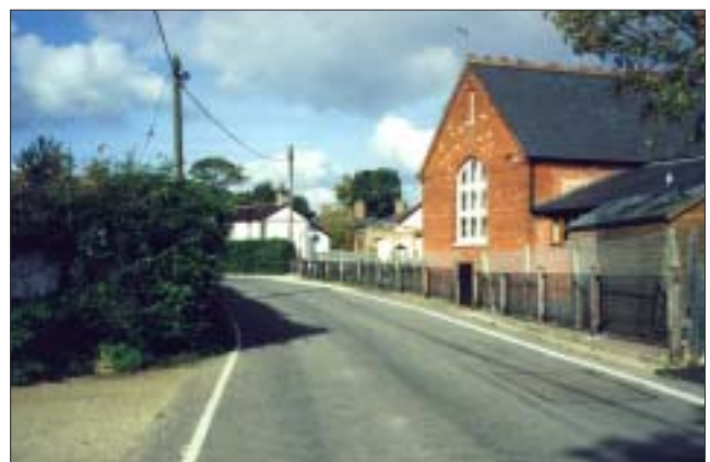
Figure 47 Edge lining on Mill Road leading to the feature illustrated in Figures 44 and 45, looking north-west (school on right). The central village speed monitoring position was in the foreground
