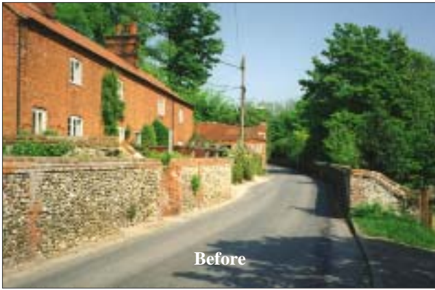
Figure 7 Stiffkey: Narrow section within 20 miles/h speed limit (eastern end just beyond the bend). Before scheme installation sections narrower than 5.5m had no centre markings. (inset: 20 miles/h repeater on wooden post.)
