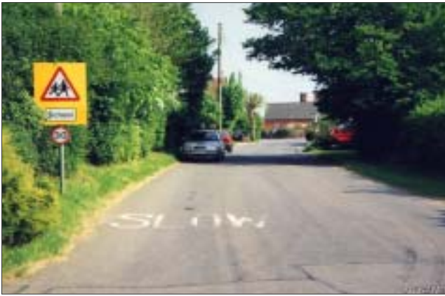
Figure 41 Patch of light coloured surfacing with edge markings on The Street to the north-west of the school (seen in distance)
