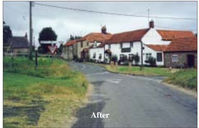
Figure 30 Wiveton: Village green, looking west from Bridgefoot Road towards C599 (ahead). Direction signing replaced by finger post arrangement; smaller 'give way' sign; wooden marker posts replacing chevron
