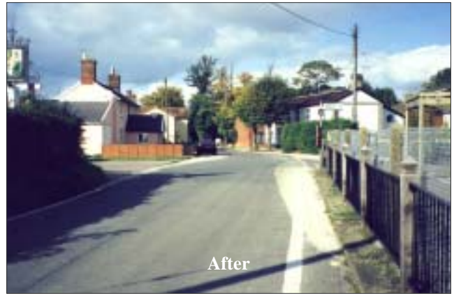
Figure 44 Light coloured surfacing laid towards e of the carriageway on Mill Road imparting horizontal deflection to traffic passing the school on the right (seen from south-east). The pub car park on the left is sometimes used for setting down and meeting children from the school
