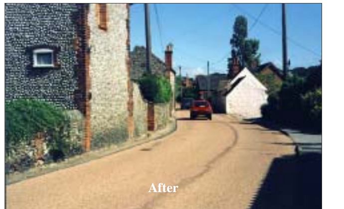
Figure 6 Stiffkey: Contrasting surface dressing and markings not reinstated within the 20 miles/h limit (looking east)
