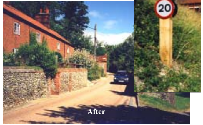
Figure 7 Stiffkey: Narrow section within 20 miles/h speed limit (eastern end just beyond the bend). Before scheme installation sections narrower than 5.5m had no centre markings. (inset: 20 miles/h repeater on wooden post.)
