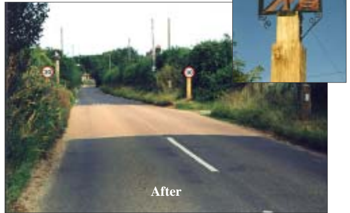
Figure 4 Stiffkey: East gateway (top) and west gateway (above). A wooden reflector post was installed on the verge and a village sign (inset) was erected just inside each gateway
