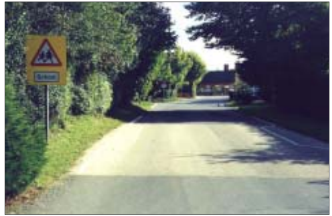
Figure 41 Patch of light coloured surfacing with edge markings on The Street to the north-west of the school (seen in distance)
