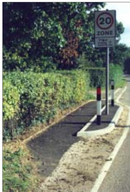
Figure 40 Detail of signing and buildout at entry on Mill Road (left) and north-west of the village centre on The Street (right)
