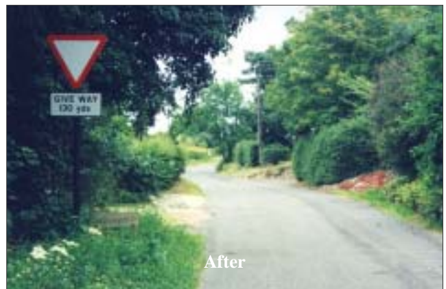
Figure 18 Blakeney: 1200mm advance 'give way' sign (left) replaced by 600mm sign, Saxlingham Road approaching A149
