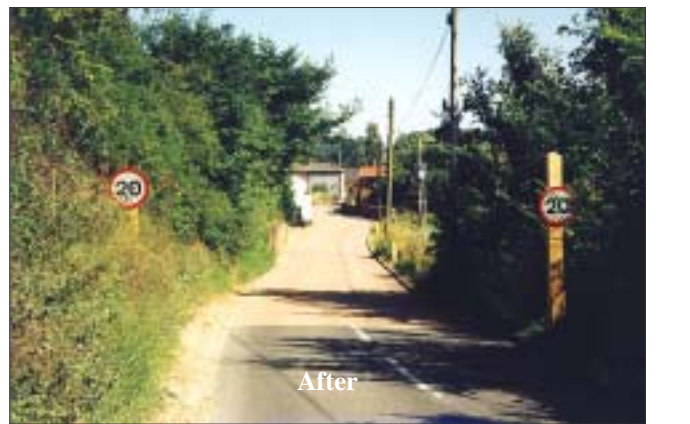
Figure 5 Stiffkey: Western end of 20 miles/h speed limit. A 'pedestrian' warning sign is on the reverse of the right hand post
