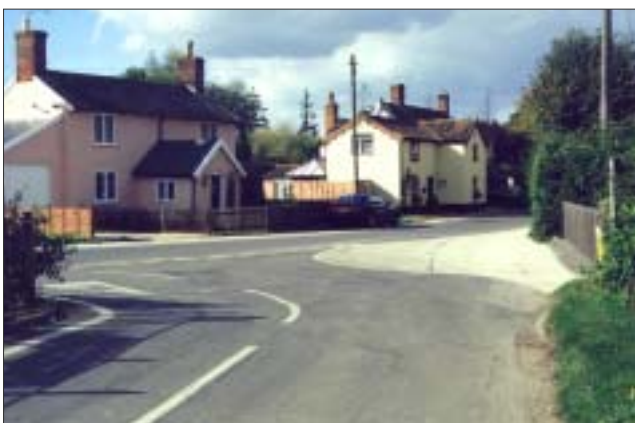
Figure 46 Alterations to the geometry of the junction of The Street and Mill Road adjacent to the school. The Street runs from the foreground to the right
