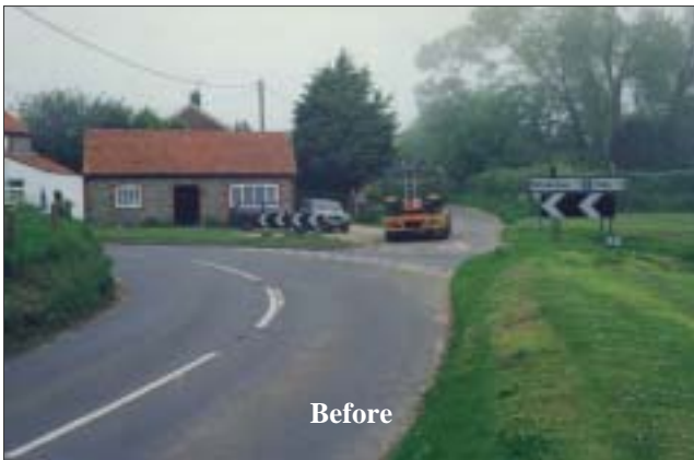
Figure 29 Wiveton: Village green, looking north along C599 (bending left) towards The Street (going ahead). Direction signing replaced by finger post arrangement; one chevron reduced in size and the other replaced by wooden marker posts
