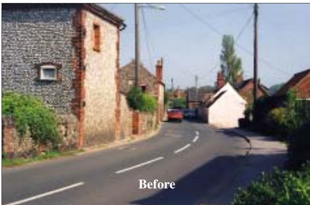
Figure 6 Stiffkey: Contrasting surface dressing and markings not reinstated within the 20 miles/h limit (looking east)
