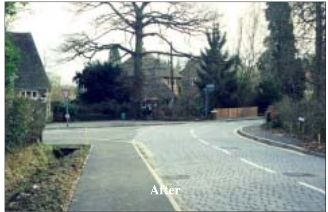
Figure 14 The junction of Norwood Hill Road (left), Rectory Lane (foreground) and The Street (right) – change of priority. The imprinted surfacing and the widened footway are also seen. Village hall on left
