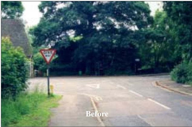
Figure 14 The junction of Norwood Hill Road (left), Rectory Lane (foreground) and The Street (right) – change of priority. The imprinted surfacing and the widened footway are also seen. Village hall on left
