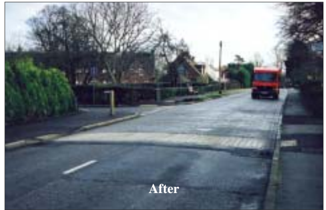
Figure 20 Similar treatment to above at the junction of The Street and Chapel Road (looking east). Footway widening and verge (by repositioning kerb) on left
