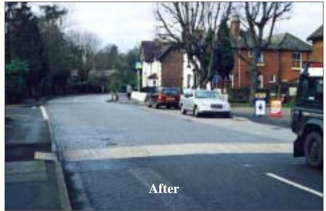
Figure 19 Imprinted surfacing shown in Figure 17 extended across junction of The Street with Ifield Road, with additional informal pedestrian crossing in foreground (looking west). Shops on the right
