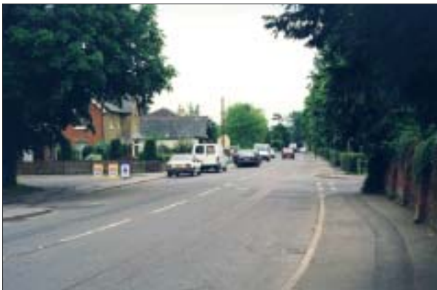
Figure 16 The Street – shops, looking east (before scheme installation). The informal pedestrian crossing was installed in the foreground
