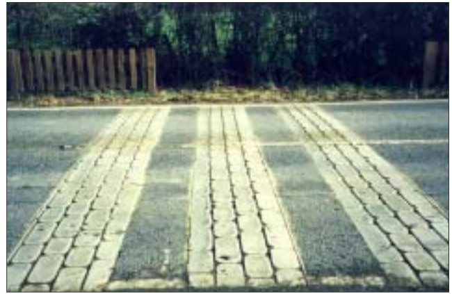
Figure 11 Northwood Hill Road – rumble strip detail
