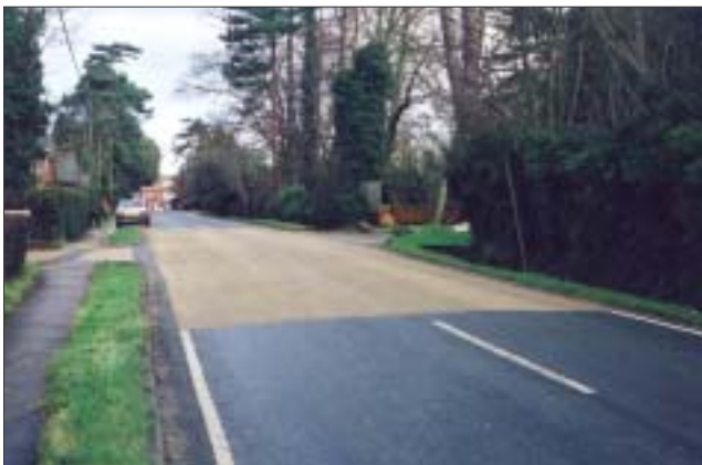
Figure 21 Imprinted surfacing, looking east, at the junction of The Street / Horley Road and Lowfield Heath Road (on right). Widened footway and renewed kerbing on right
