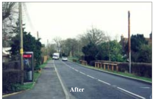
Figure 13 Horley Road, looking east – widened footway with granite kerbs replacing concrete; fencing on right. The camera position is at what would have been the eastern end of the 20 miles/h speed limit, but extension of the imprinted surfacing to this point (just east of the Lowfield Heath Road junction) commenced in September 2000
