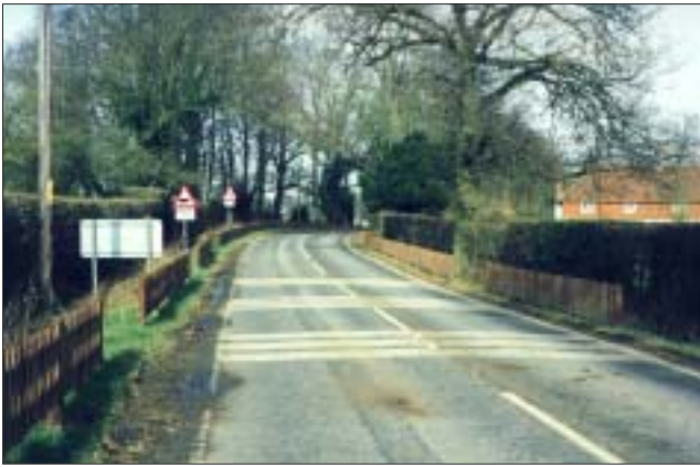
Figure 10 Northwood Hill Road – rumble strips and fencing looking north towards gateway round bend
