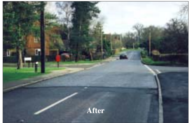
Figure 21 Imprinted surfacing, looking east, at the junction of The Street / Horley Road and Lowfield Heath Road (on right). Widened footway and renewed kerbing on right
