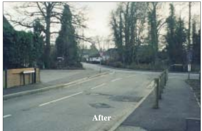
Figure 15 As Figure 14 but from Norwood Hill Road, looking towards village centre. The After photograph shows the kerb build-out (left), footway widening and timber reflector posts
