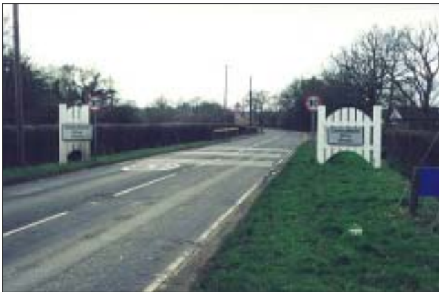
Figure 5 Horley Road, with rumble strips of the imprinted material used within the village
