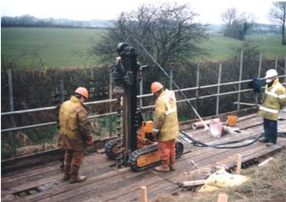
Plate 2 Drilling rig operating on a platform
