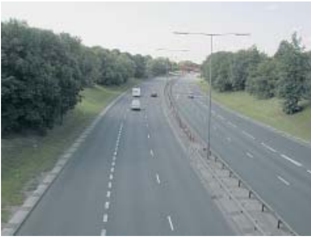
Figure 5.10 Site H (the left carriageway) BOS slag sections
