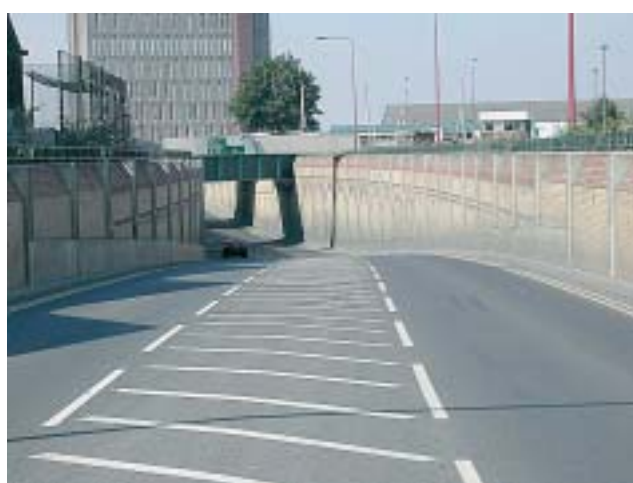
Figure 5.8 Site G: underpass section looking north
