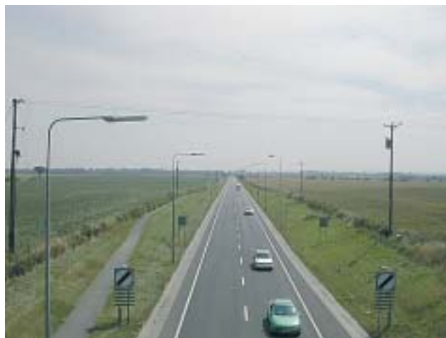
Figure 5.6 Site G: de-restricted section looking south
