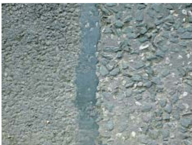
Figure 5.3 The surfacings on site D (BOS slag SMA to the left)
