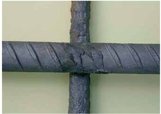
Figure 4.5 Example of corrosion of longitudinal and transverse bars
