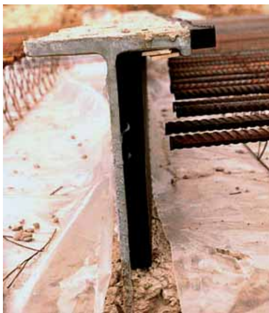
Figure 8.1 The wide-flange beam system
