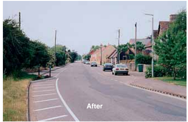
(a) Removal of centre lining within village. Also shown: hatching between sough gateway and first build-out, with new parking bay beyond
