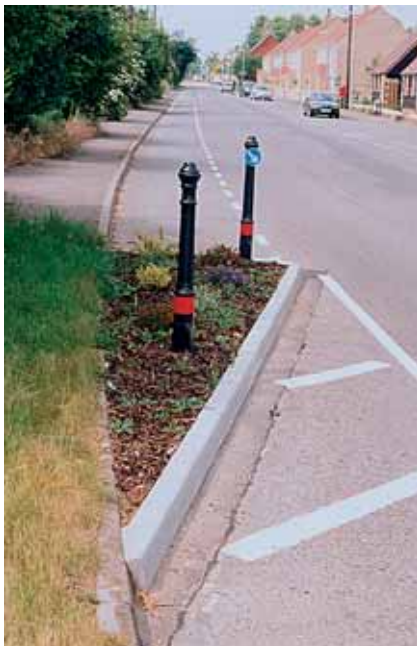
(c) Build-out with parking bay beyond
