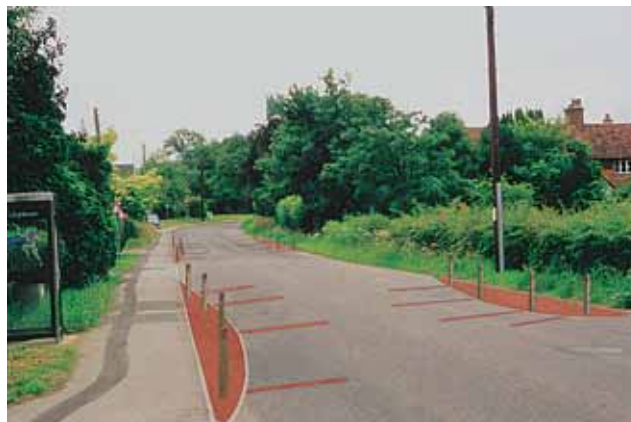
5: Build-outs with posts, lines on road surface, no centre line
