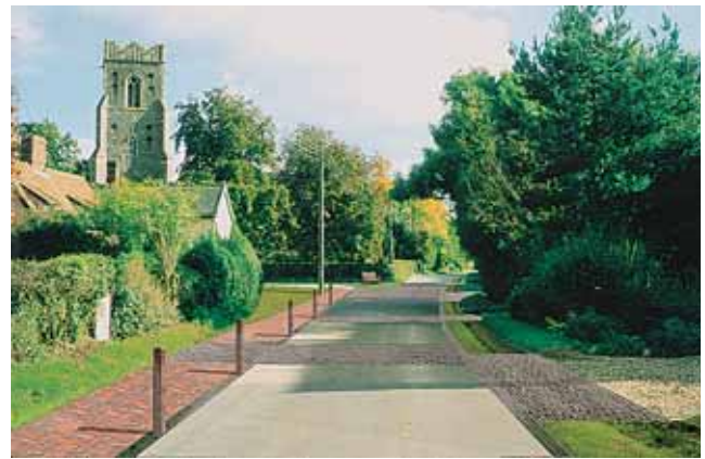
4: Footway and driveways
