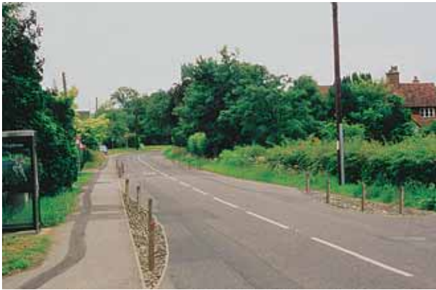
3: Build-outs with posts, centre line
