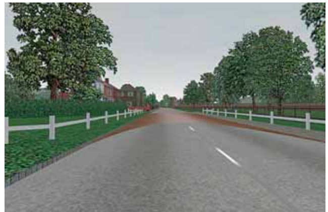
Curved patch (excessive camber) (V6)
