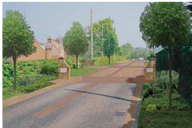
5: Gateway and continuous coloured surface with patches
