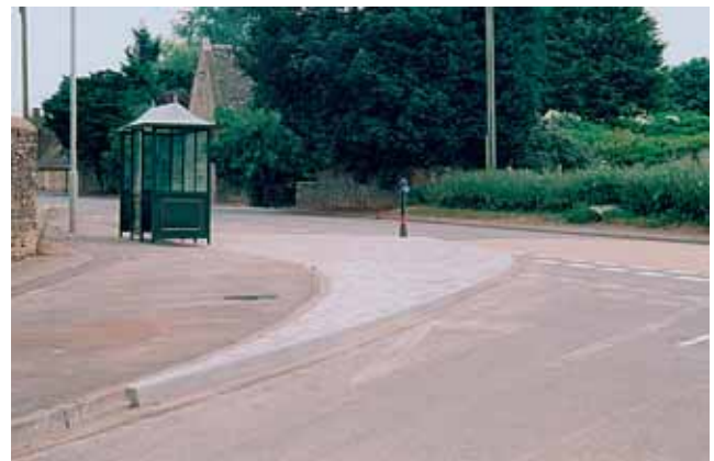
(e) Paved build-out at the junction with Gosditch
