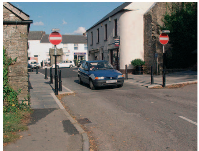
Figure 3.20 No entry at southern end of home zone
