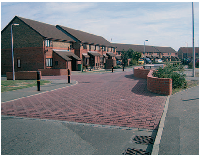
Figure 3.13 Chicane and bollards at spur cul-de-sac junction looking east
