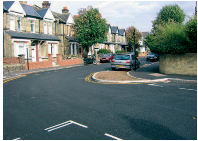
Figure 3.38 Build-out on bend, sheltering new parking bays each side of build-out, Hastings Road (looking east)
