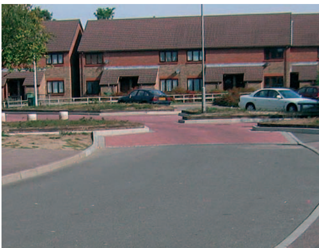
Figure 3.14 View of new road layout near Roentgen House looking north
