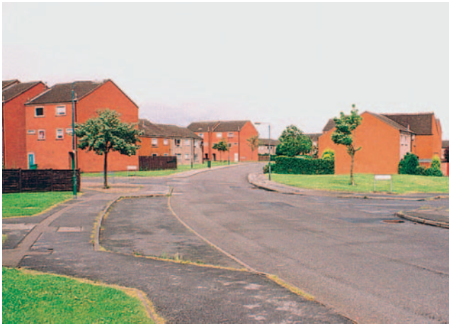
Figure 2.13 Nobel Road, middle section, near Park Gate Community Centre, looking north, before the home zone was installed
