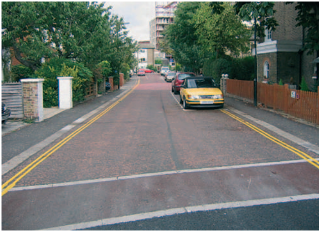
Figure 3.36 Shared surface, Denmark Road
